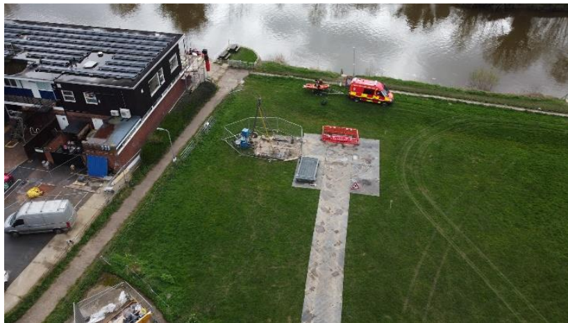
Ground Investigation at the Rowing Club. Photo taken on 6 March 2024
