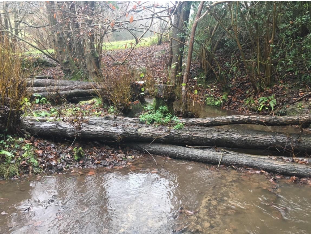
Figure 2-7: Example Semi-Natural Large Woody Debris Structure
