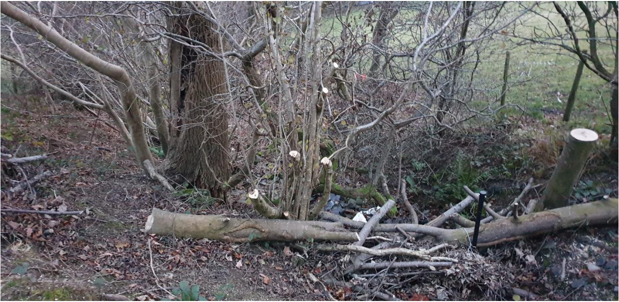
Figure 2-6: Example Gully Blocking with Woody Debris
