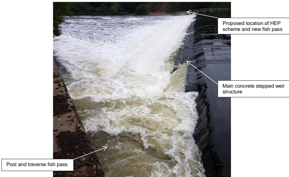
Figure 1-1. Gunthorpe Weir looking towards the right/eastern river bank on 05 June 2018.
