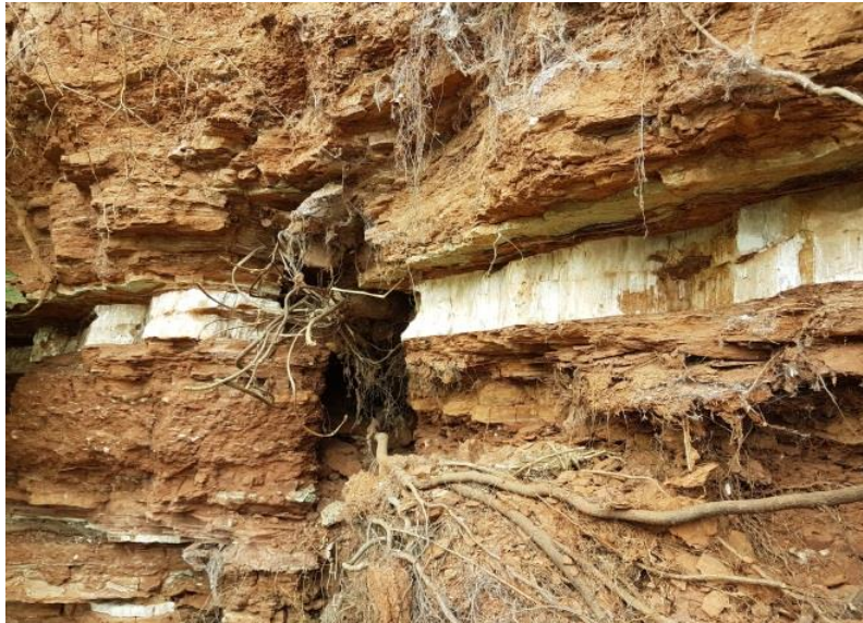
Figure 3-4. Cliff face material on the right bank downstream of Gunthorpe weir.
