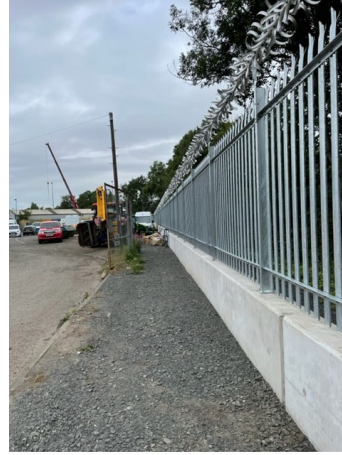
Photo 2 Tyne Mills flood wall
