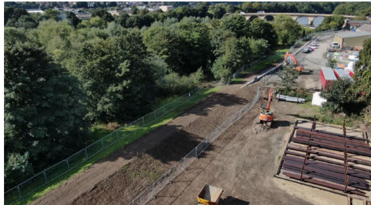
Photo 4 Bridge End embankment
