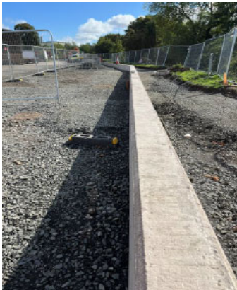
Photo 3 Bridge End flood wall
