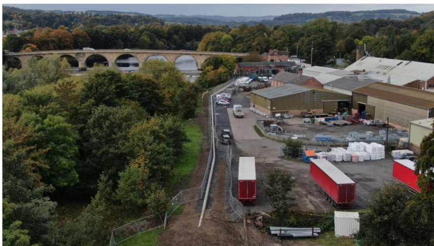
North bank flood wall and embankment
