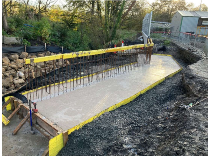
South bank flood wall
