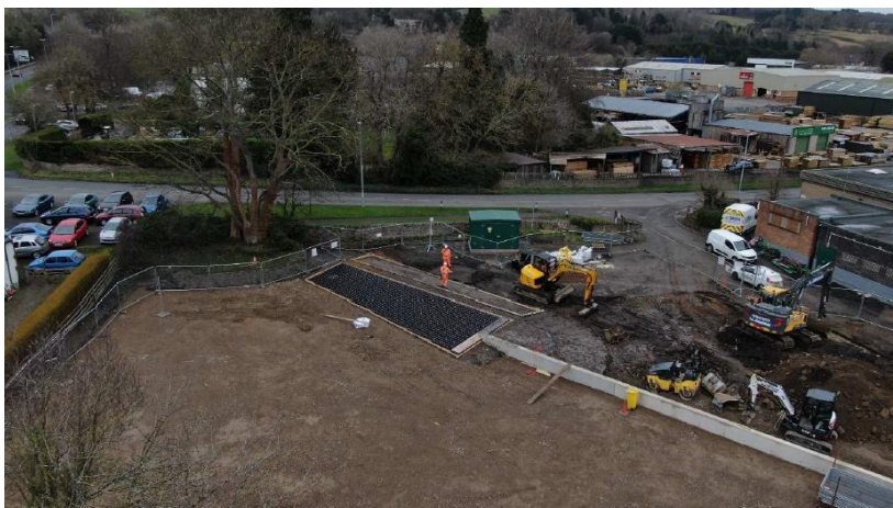
North bank flood wall and embankment
