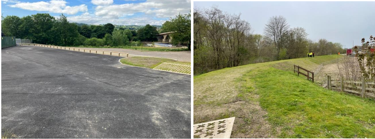
North bank flood wall and embankment
