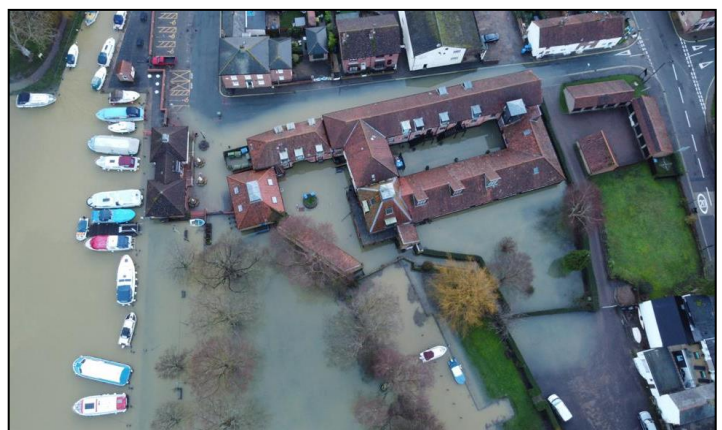
Flooding at Fen Lane and the Quay in Beccles, December 2020. Photo credit Paul Rudland https://alldrone.uk/ .
