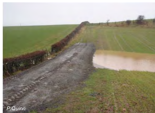
Bunds across known surface water flow paths to retain runoff and sediment. This bund acts as a track, elevated above the saturated ground, enabling access to the rest of the field and providing an additional benefit for the farmer.
