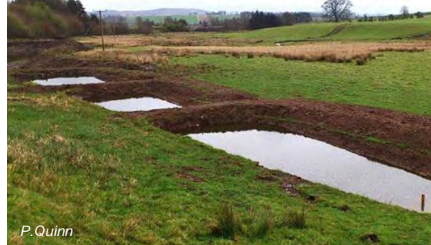
Series of offline ponds that also act as sediment traps.
