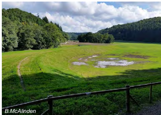
Bund at Newbridge providing flood storage
