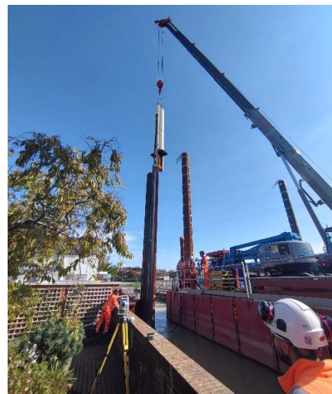
Photo of installation of sheet pile
