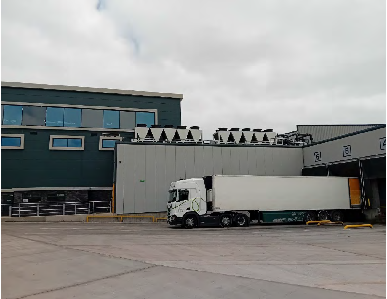
Plate 1 VIEW OF SITE SURFACING
