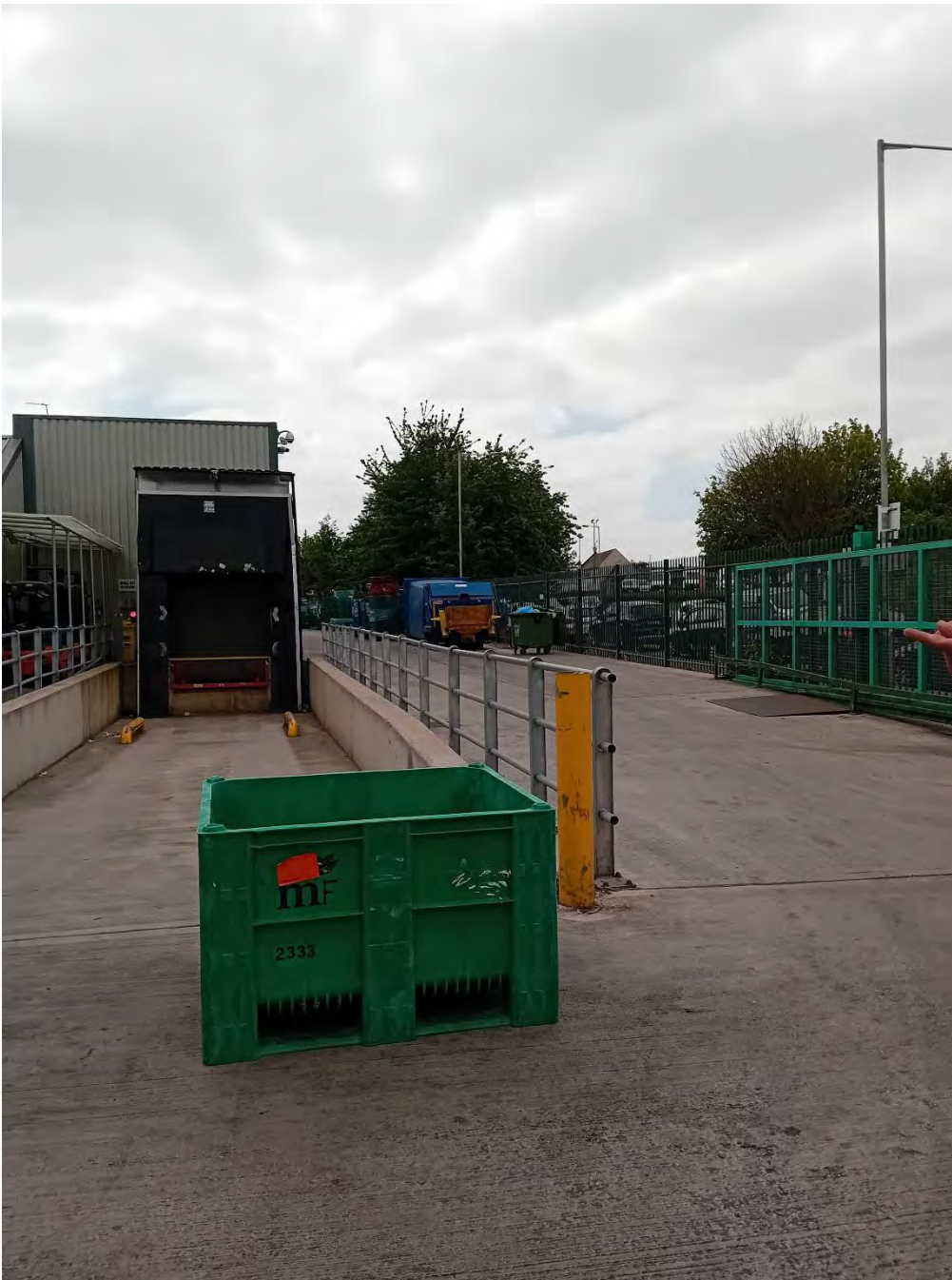
Plate 2 MATERIAL INTAKE AREA
