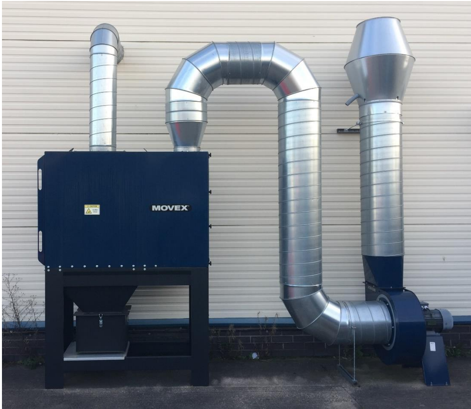
Typical CFE Filter Installation
