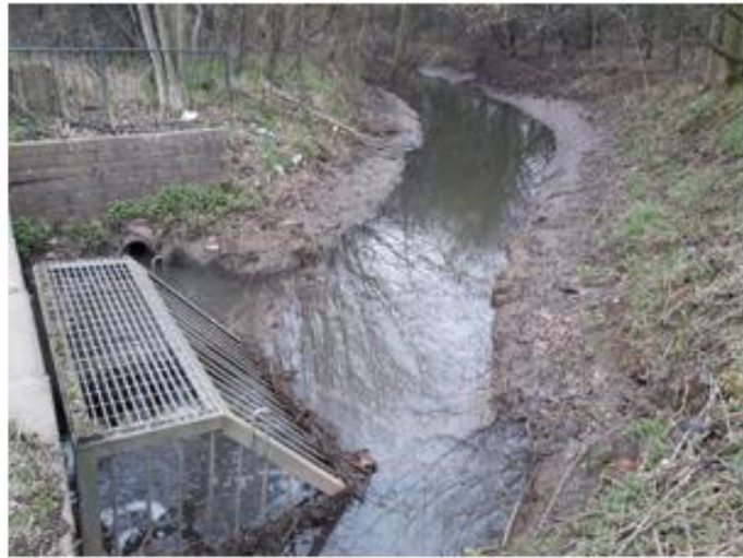
Drain with flow from "Brick Kiln Pool" area at Culvert with Stubbers Green Road. Headwall and secondary inflow from ditch adjacent to the roadside verge which continues towards the roundabout. View Northwest.
