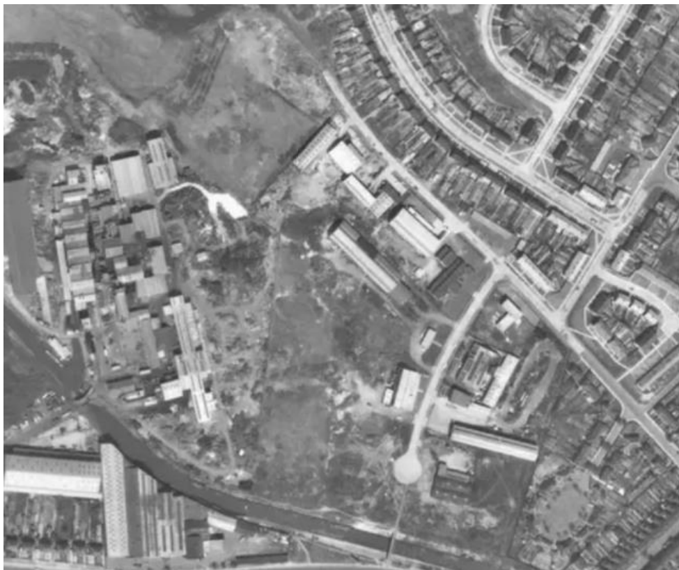
Aerial Photo - raf_543_2336_v2_0119 July 30th 1963: https://historicengland.org.uk/
