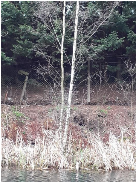
Figure 2: Hole in northern bank of canal
