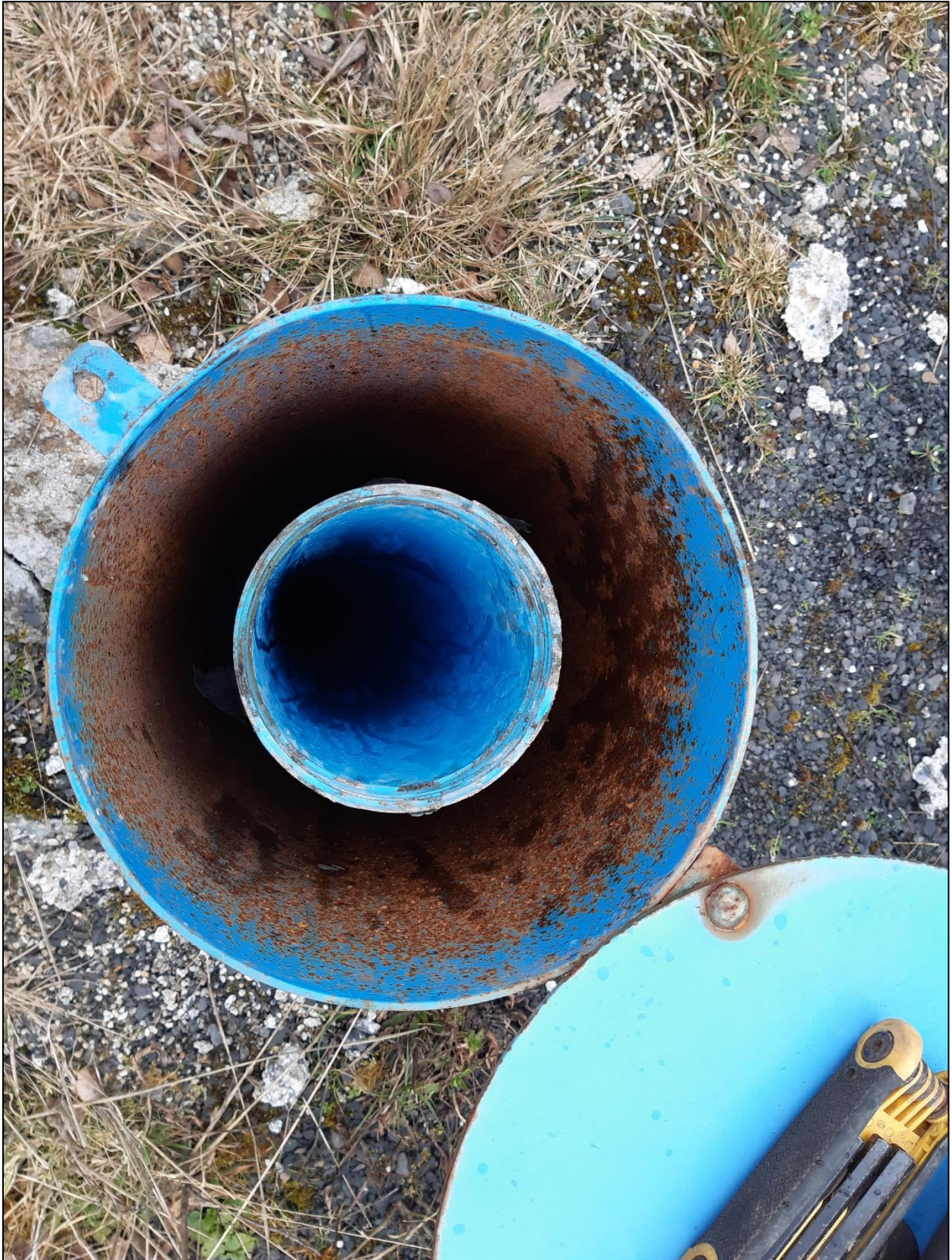
P4 – BH01-19 Installation
