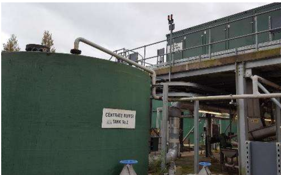
Photo 8: De watering centrifuges and centrate buffer tank
