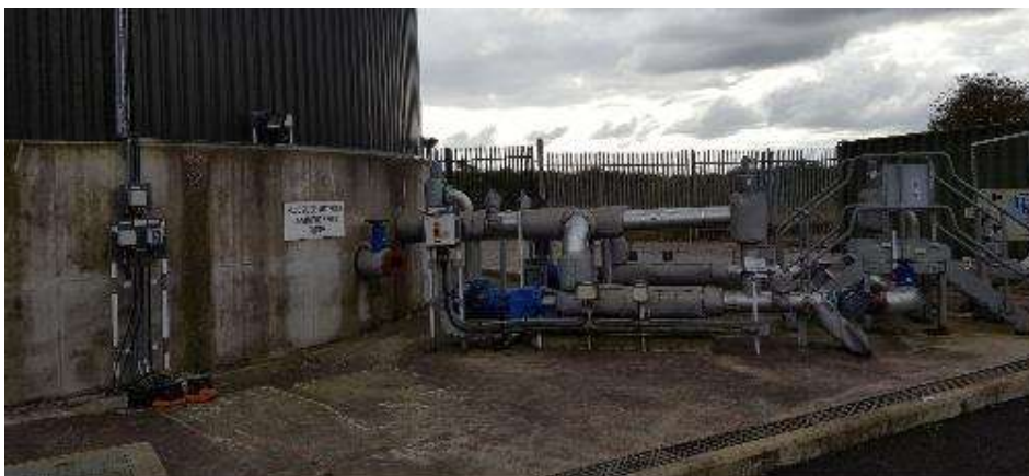
Photo 14: Impermeable surface and drainage around tanks
