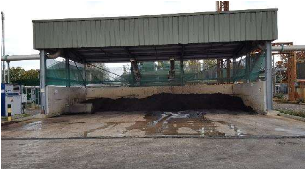
Photo 10: Cake storage building
