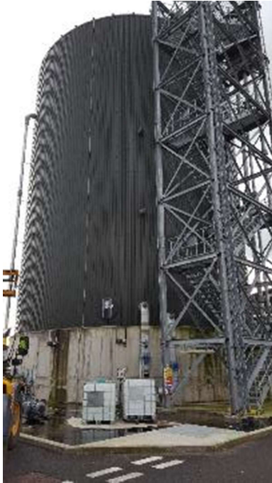
Photo 5: Anaerobic digester
