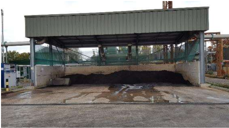
Photo 1: Cake storage building
