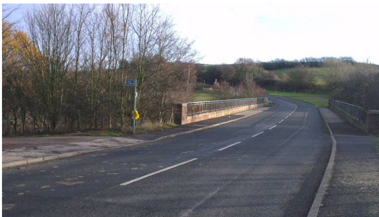
View east across road bridge with existing lay-by junction
