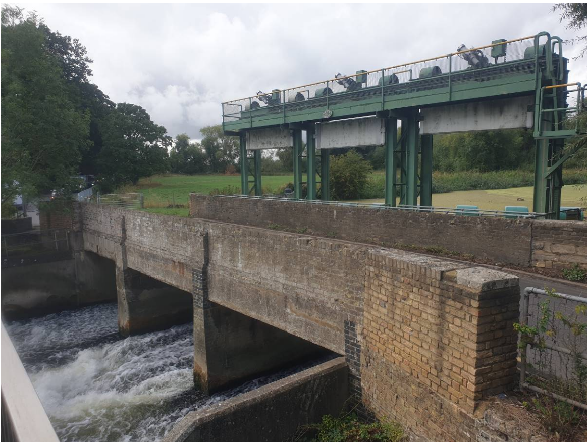
Figure 8: EA sluices – view to proposed site, across road bridge, from footway
