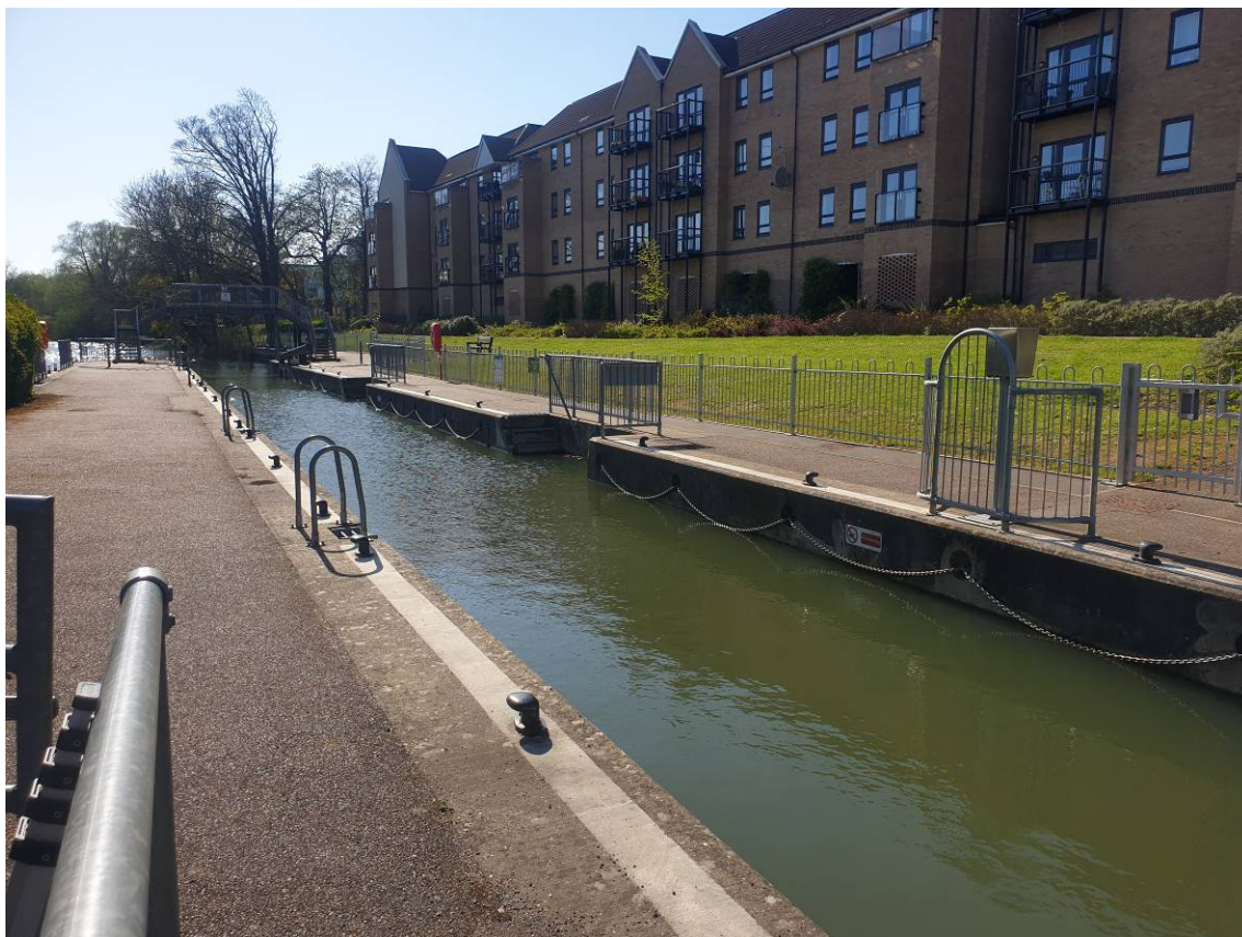
Figure 13: Navigation branch – lock, viewed upstream (no impact)
