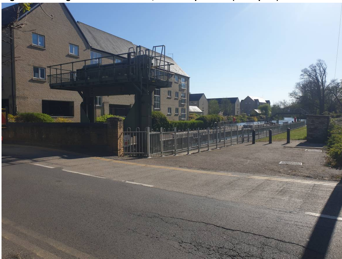
Figure 14: Navigation branch – bridge and lock downstream gate, viewed upstream
