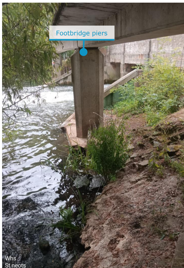
Figure 11 Downstream of Mill Lane sluice
