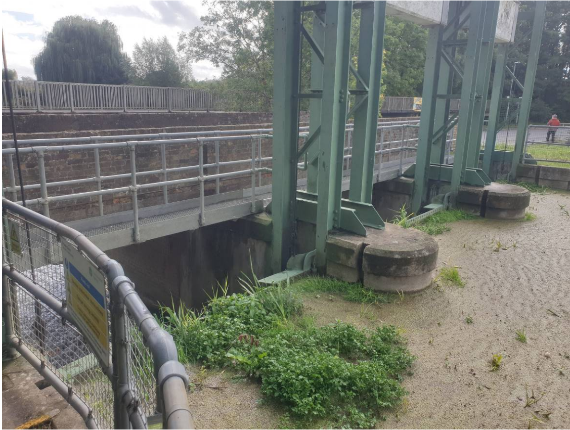
Figure 3: EA sluices – view downstream from north bank, with bridge and footway
