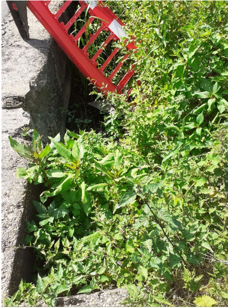
The roadside ditch
