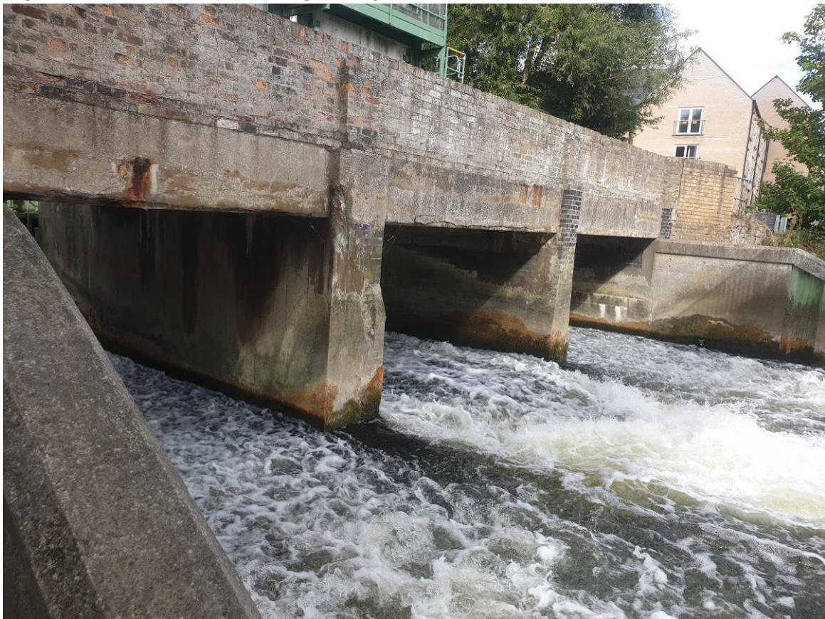
Figure 10: EA sluices – discharge splay, view across from south bank of sluices
