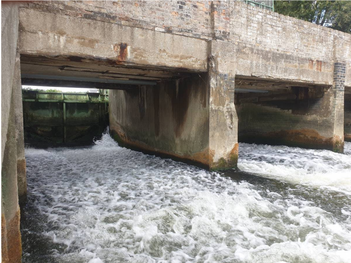
Figure 9: EA sluices – discharge splay, view upstream from south bank of sluices
