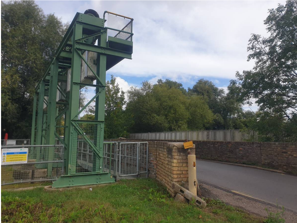
Figure 5: EA sluices – view from site on south bank, with bridge and footway
