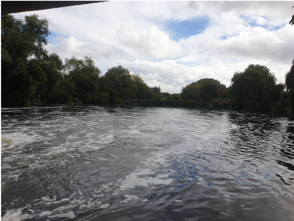
Figure 12: EA sluices – tailwater pool, view downstream from south bank of sluices
