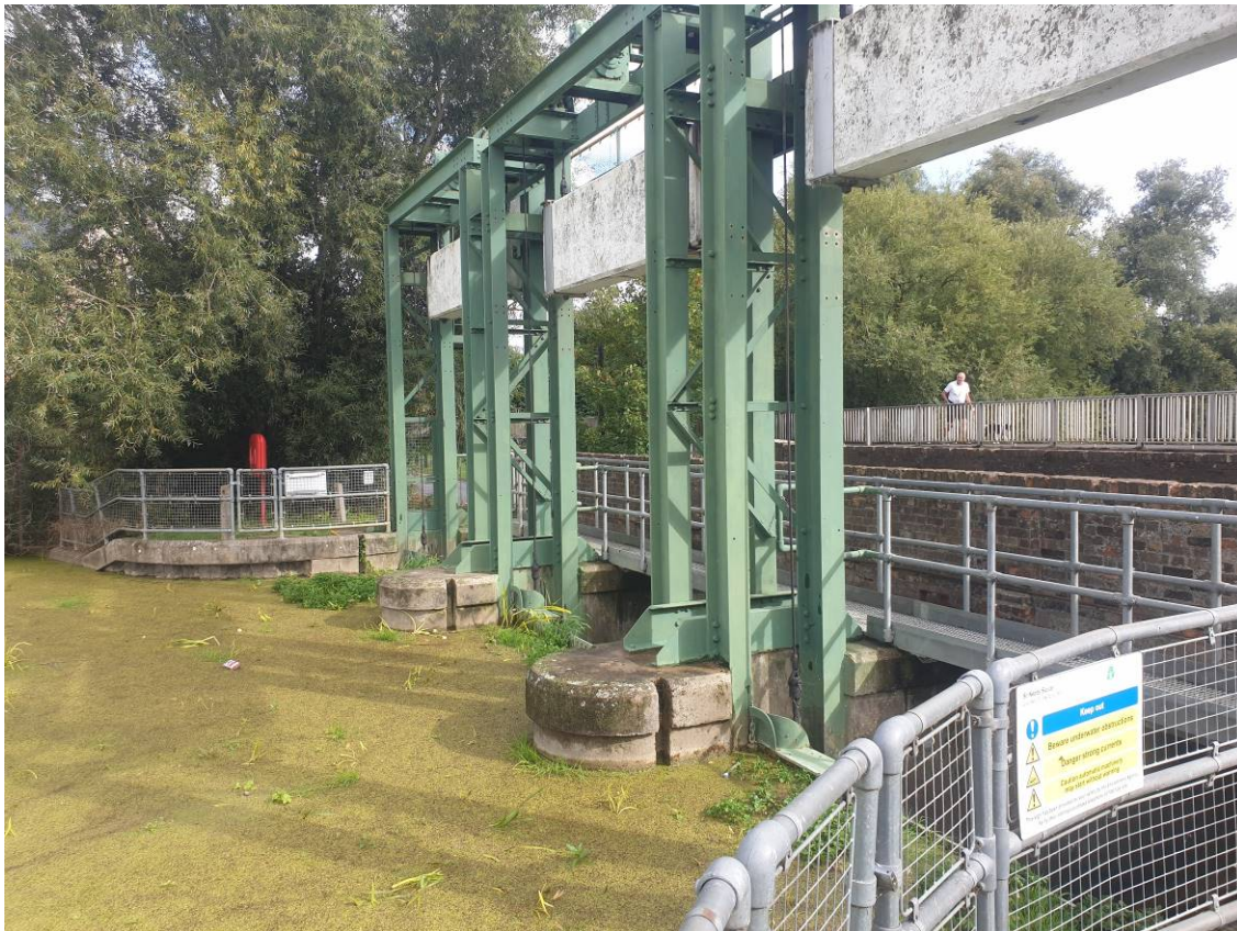
Figure 4: EA sluices – view downstream from south bank, with bridge and footway
