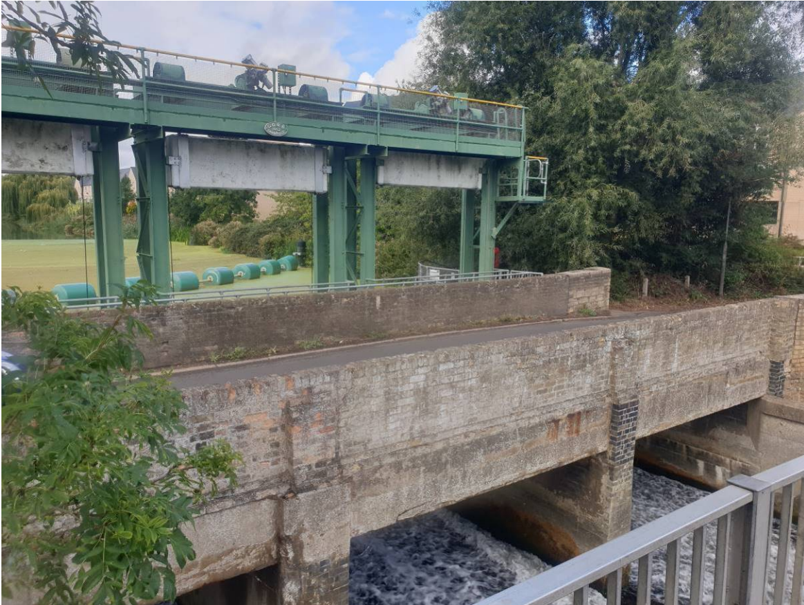
Figure 7: EA sluices – view upstream across road bridge, from footway
