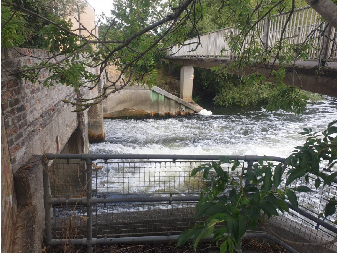
Figure 11: EA sluices – discharge viewed from south / from proposed new discharge
