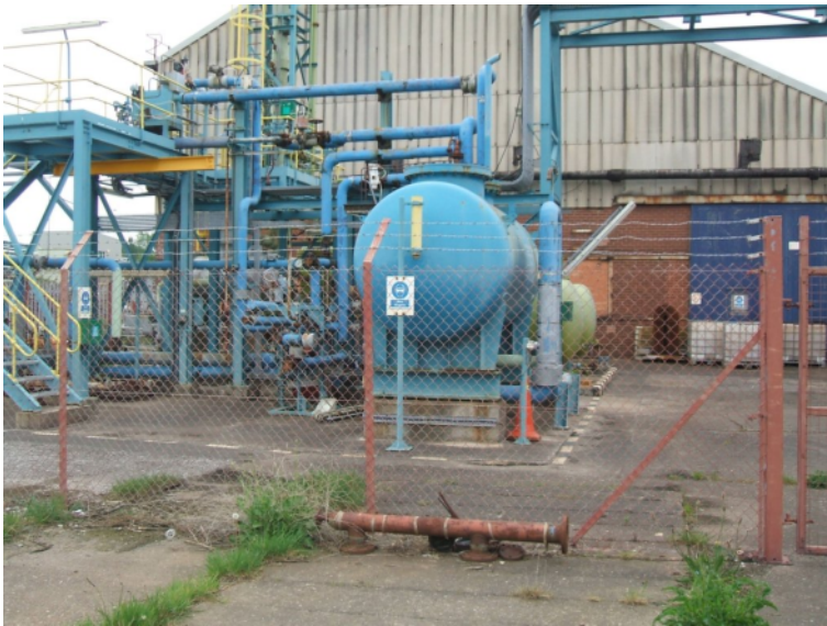
Photo 7 View of training rig located adjacent to the Weston workshop
