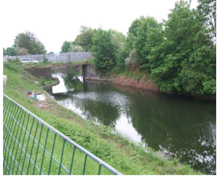
Photo 14 Runcorn Western Canal looking South
