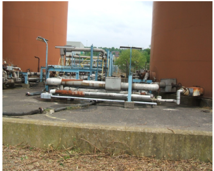
Photo 8 View within bund area of the redundant tanks
