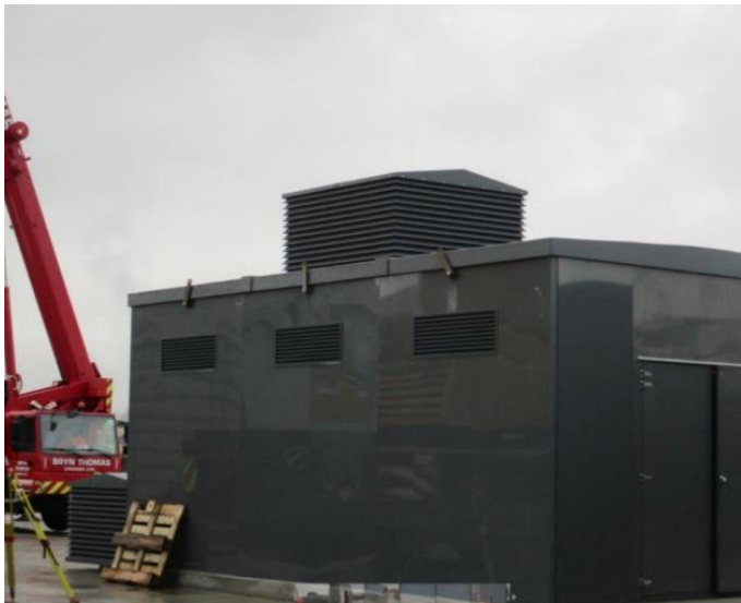
Figure 3-7 – GRP compressor enclosure photograph
