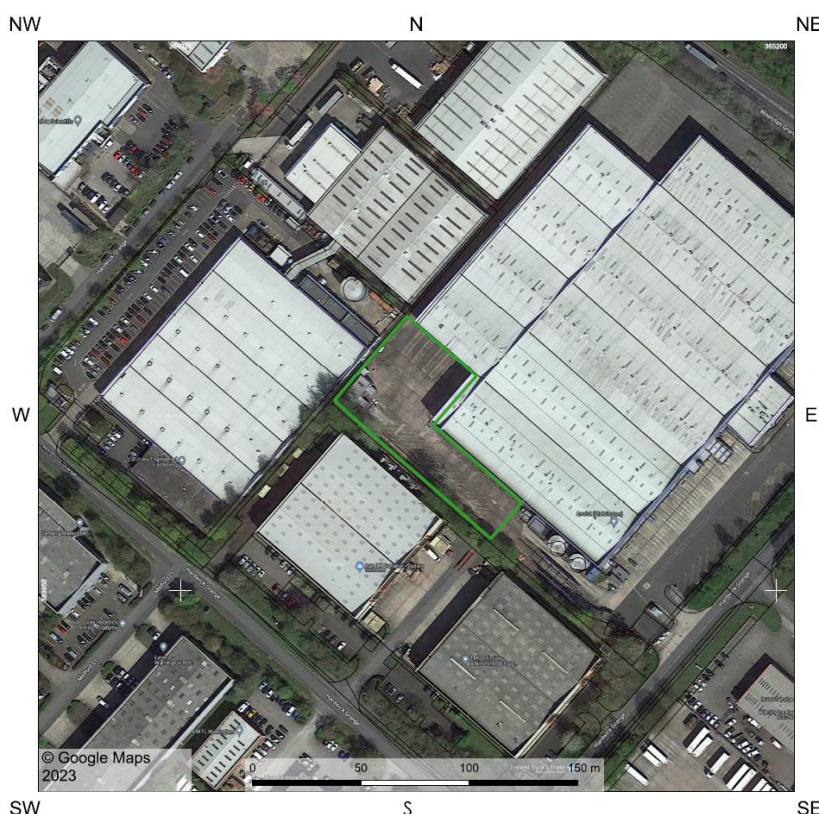
Figure 1 Aerial image of the site, showing the permit boundary in green
