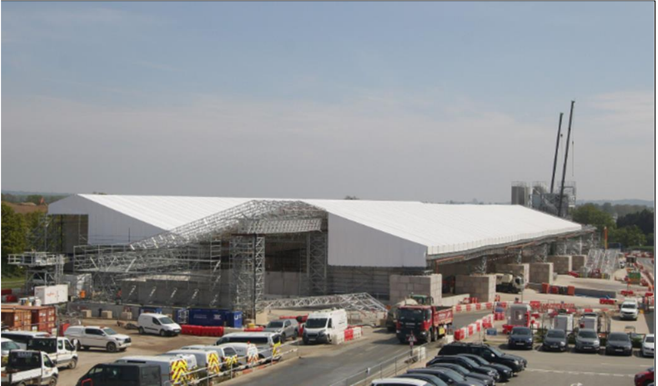
Figure 1 – STA Construction – roof installation (May 2023)
