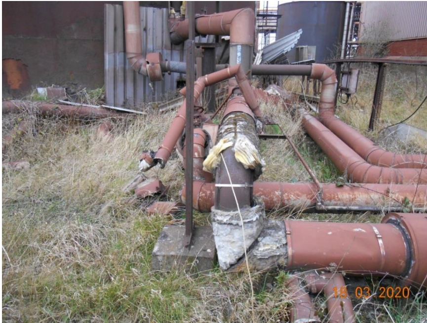
Plate 28 – Diesel tank connections and fibrous pipe lagging.
