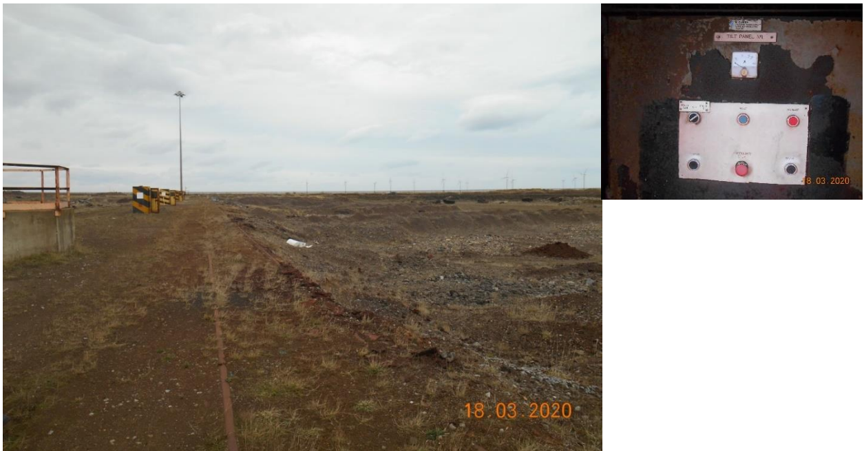
Plate 7 – View looking north west along the alignment of the steel torpedo 'pond area'. The tilt operation booths are seen yellow/black on the left hand left-hand side of the photograph (see insert showing Tilt Panel to the right), with running rails for the tippers shown on the edge of the 'pond' areas.
