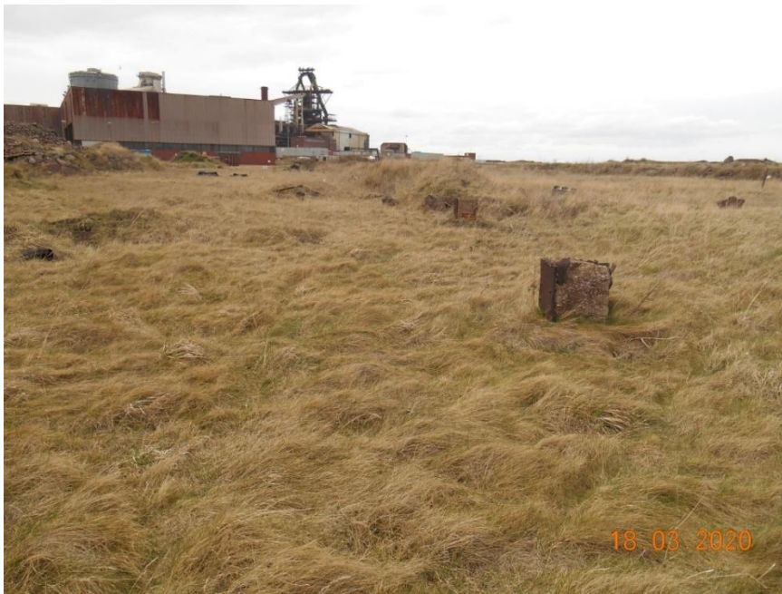
Plate 15 – View looking north west showing cut-down structure stanchions along the alignment of the former Redcar Steel and Iron works Steel Plant building.
