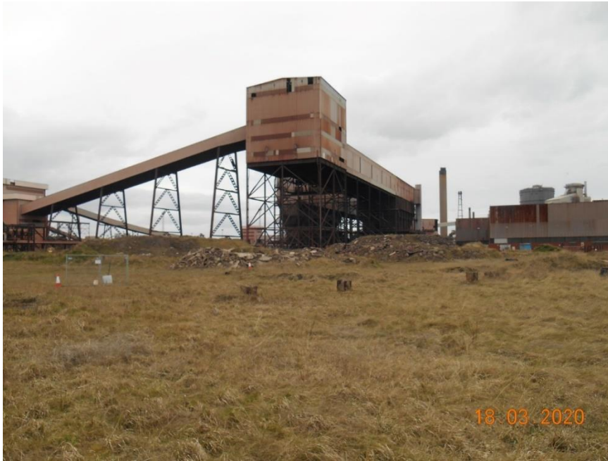
Plate 14 – View looking west showing stockpiles, former refuelling area and historical cut-down structure stanchions.
