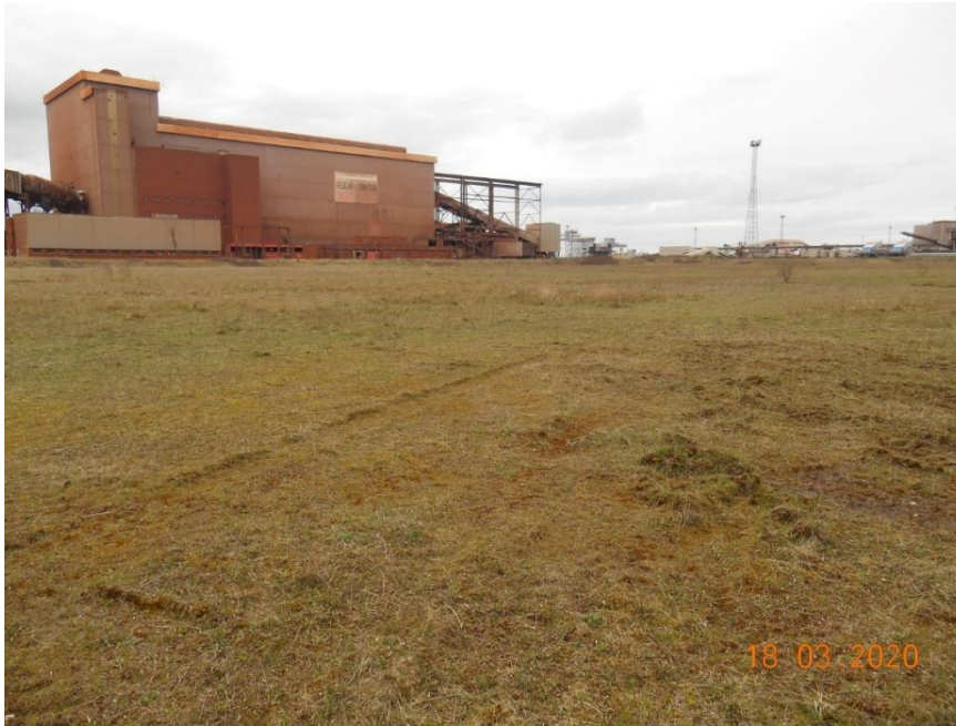
Plate 21 - View looking south west showing the Sinter Plant adjacent to the south boundary of the proposed site.
