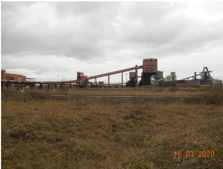
Plate 13 – View looking west showing area of open ground, Blast Furnace Stockhouse and associated buildings. The Blast Furnace is shown on the right hand side of the photograph which is outside and north west of the proposed site boundary.
