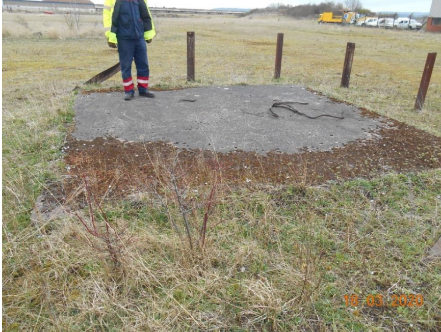
Plate 25 - View looking east southeast showing foundation base.
