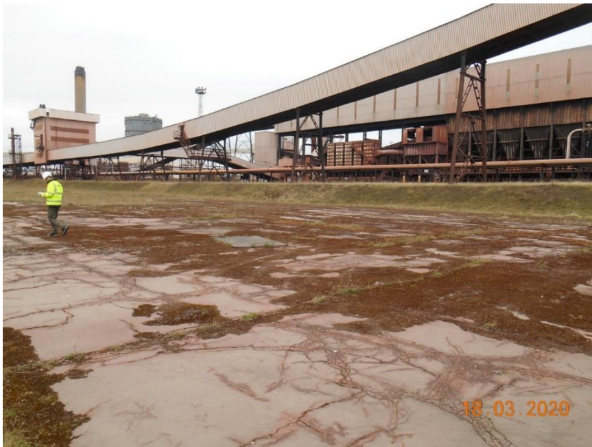
Plate 22 – View looking north west showing area of remnant hardstanding and the Blast Furnace Stockhouse.
