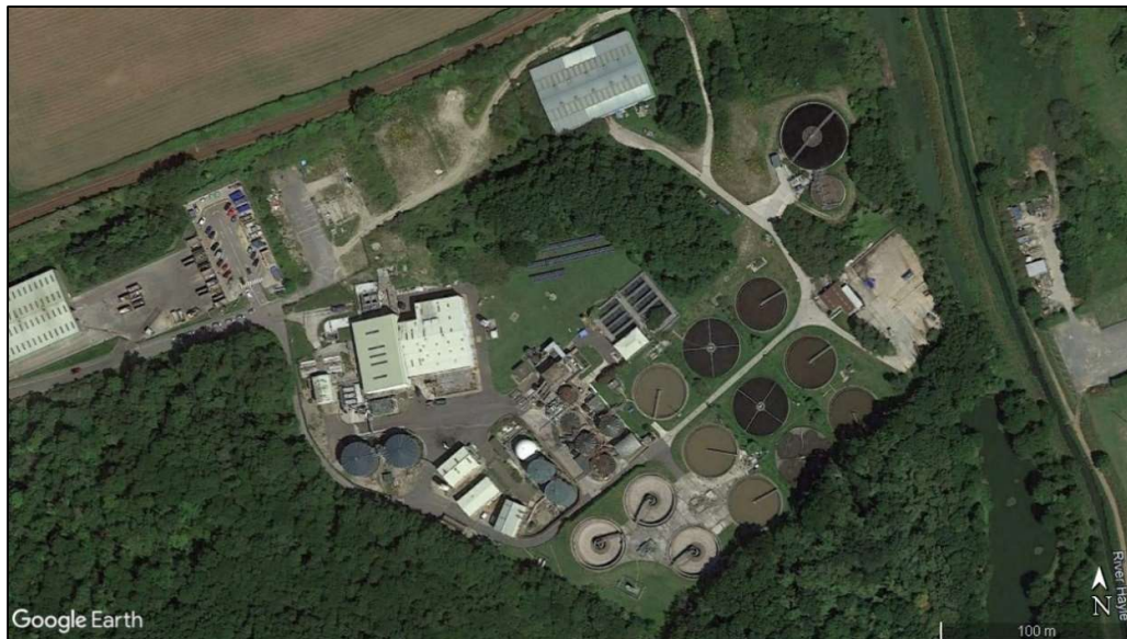
Figure 1: Hayle WWTW aerial view
