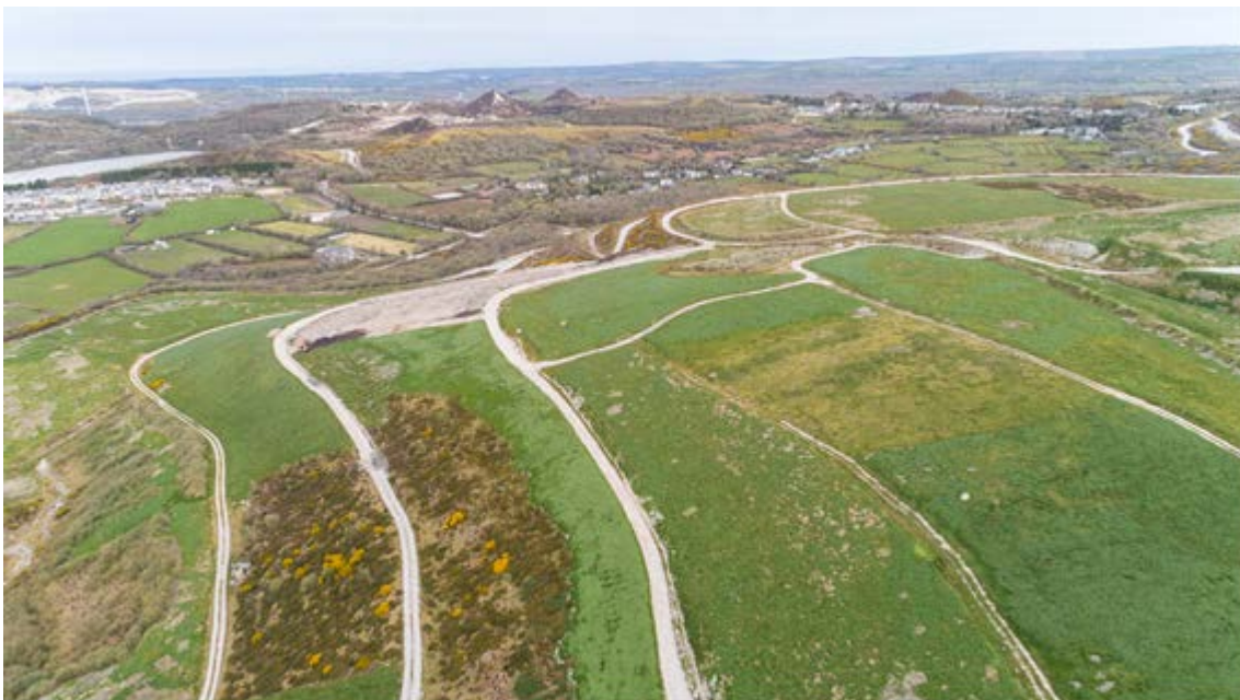
Photo 1. Example of restoration areas at neighbouring IMERYYS site at Dubbers.
