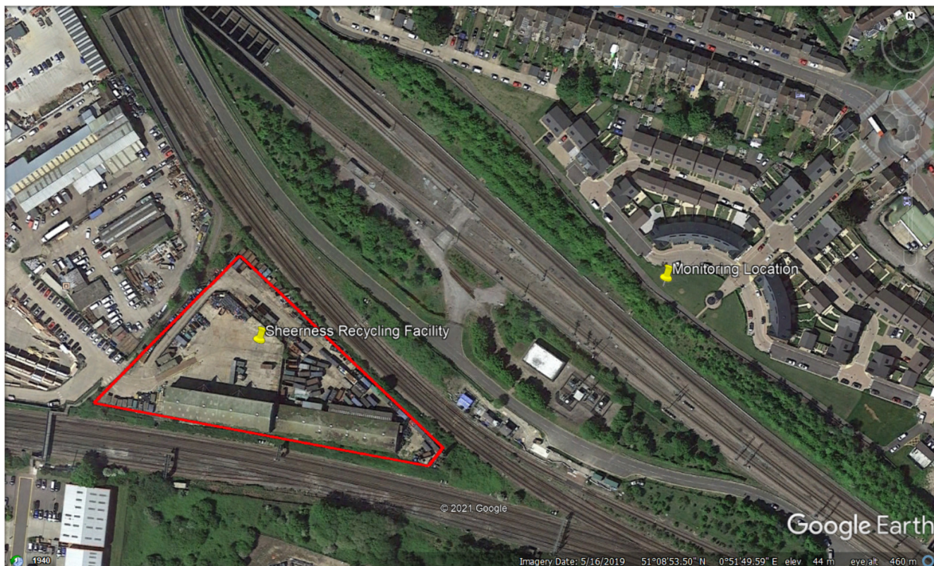
Figure 3-1 Monitoring and Nearest Receptor Location
