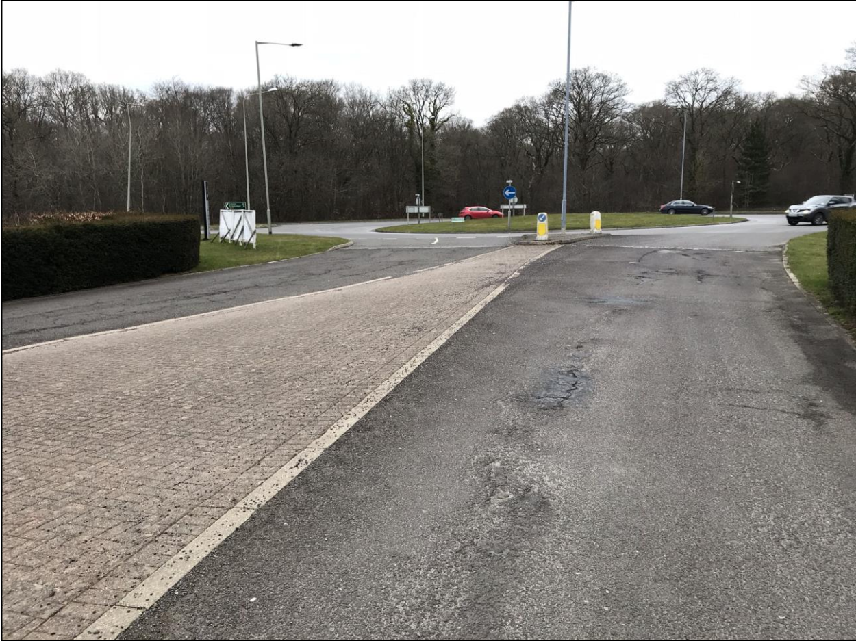
Figure 28 View of Existing roundabout at the golf club entrance
