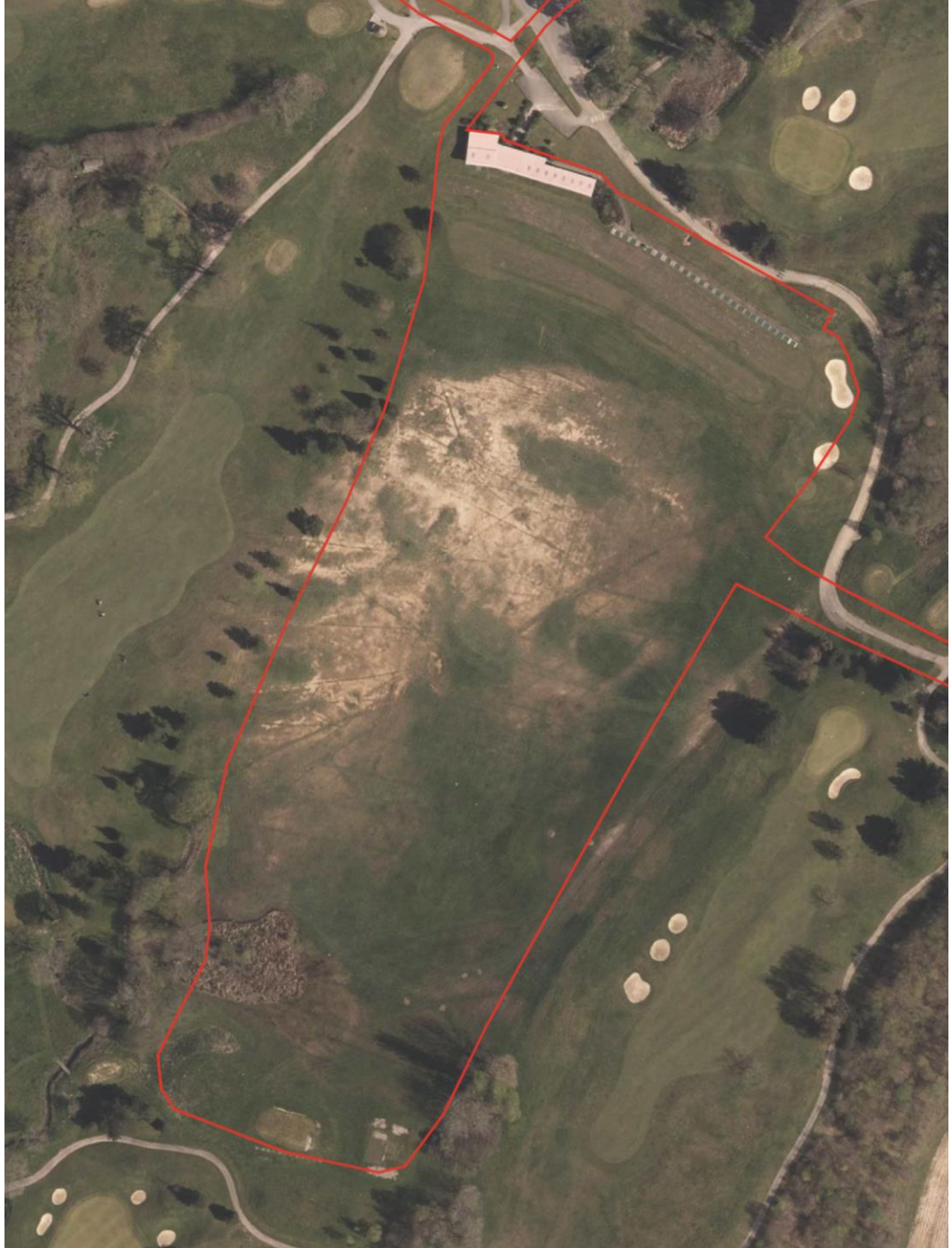
Figure 005 - Recent aerial showing extent turf (note extent of drainage lines that have failed to address the problem)
