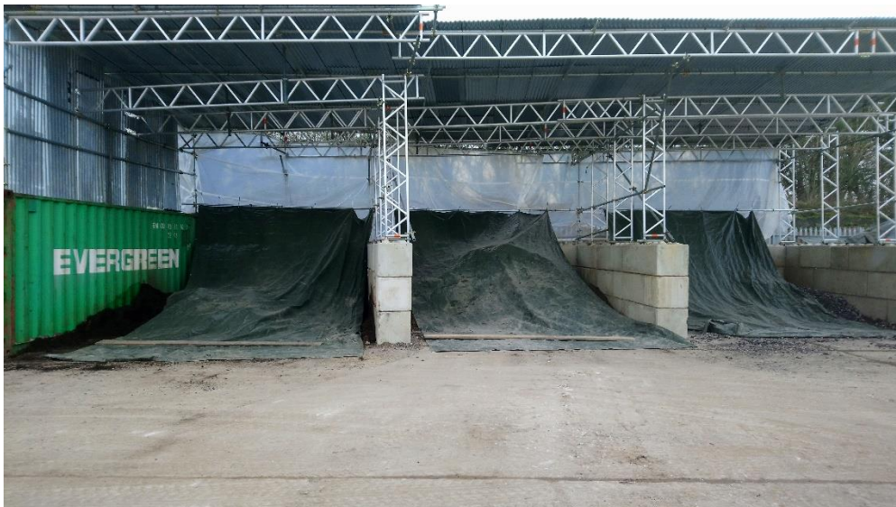
FIGURE 4.1: PHOTOGRAPH SHOWING COVERED STORAGE BAYS
