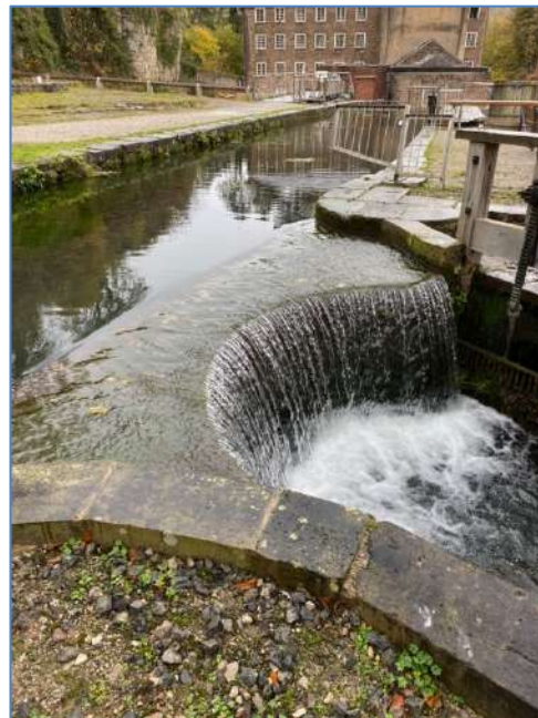
Figure 7. Headrace canal and horseshoe weir - looking east -
