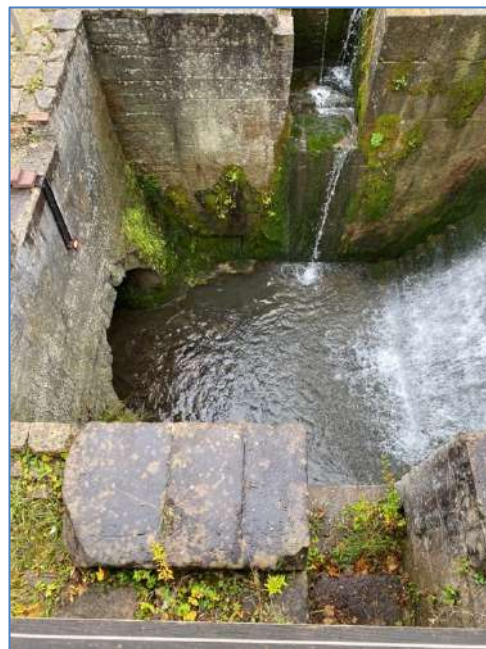
Figure 4. Wheel pit interior
