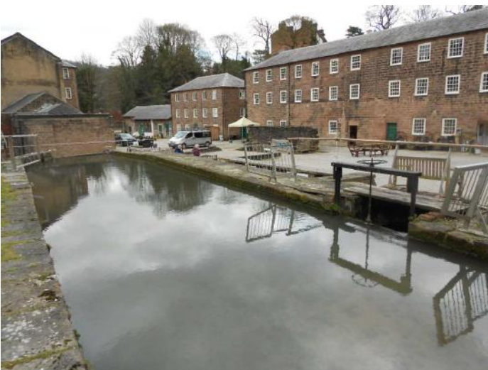
Figure 30 : Side-sluice allowing the millrace flow to be diverted away from the wheelpit
