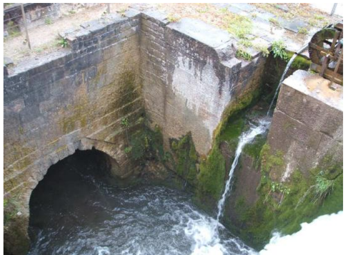
Figure 26 : Exit tunnel to the Derwent
