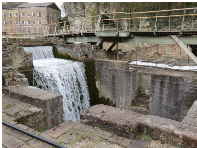
Figure 25 : Wheelpit with symmetrical bearing mounts
