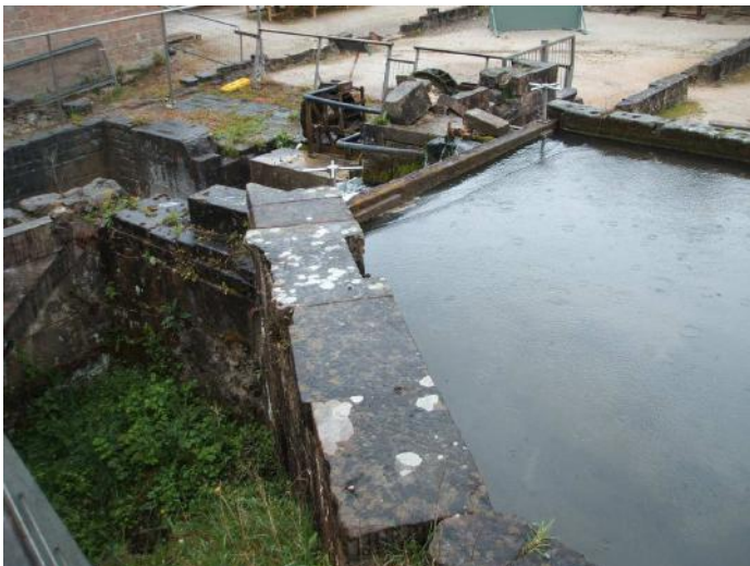
Figure 24 : Overspill with adjustable stop-log
