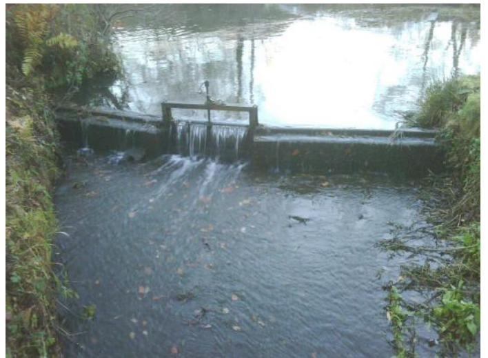
Figure 6 : Discharge over the Leawood spillway into the Derwent on 26/11/21
