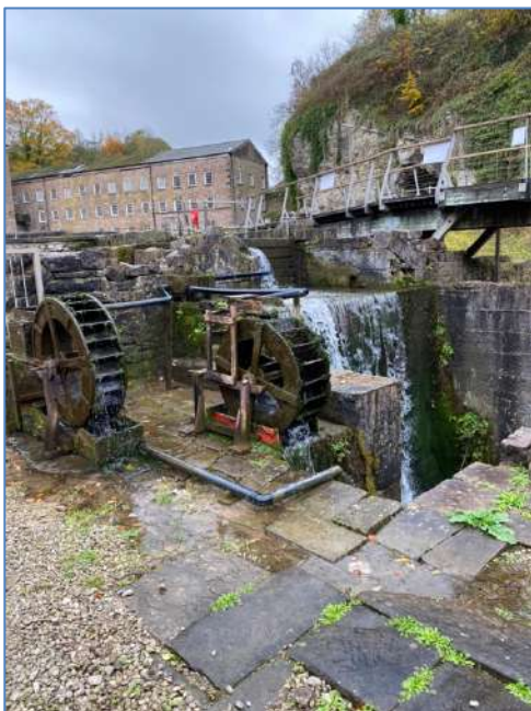
Figure 3. Wheel Pit looking north-west
