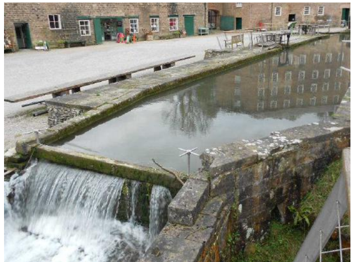
Figure 24 : Overspill with adjustable stop-log
