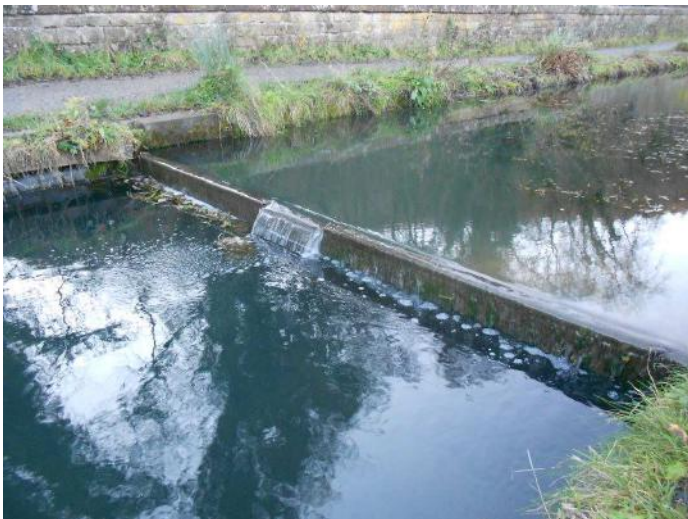
Figure 5 : Discharge over the Leawood impoundment on 26/11/21
