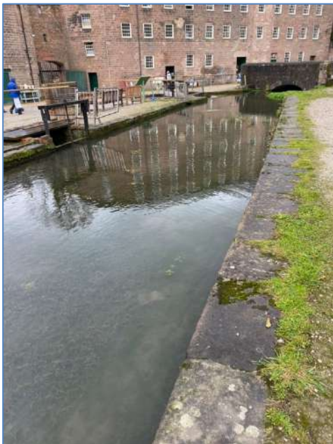
Figure 6. Headrace canal - looking west towards footbridge
