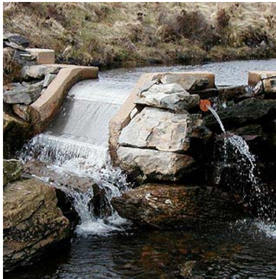
Plate 3.6 Example of a Screen B Coanda installation (Dulas Hydro)
