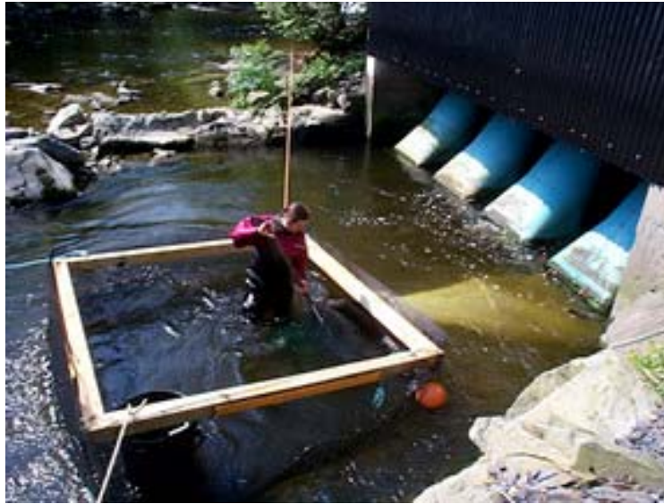
Plate 7.1 Total flow netting at the draft tube of a small hydropower turbine. Here, fish enter a live-car at the cod-end of the net to facilitate removal and to reduce the likelihood of net-induced injuries .
