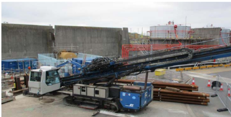
Figure 5.23 Photograph of HDD drilling rig.
