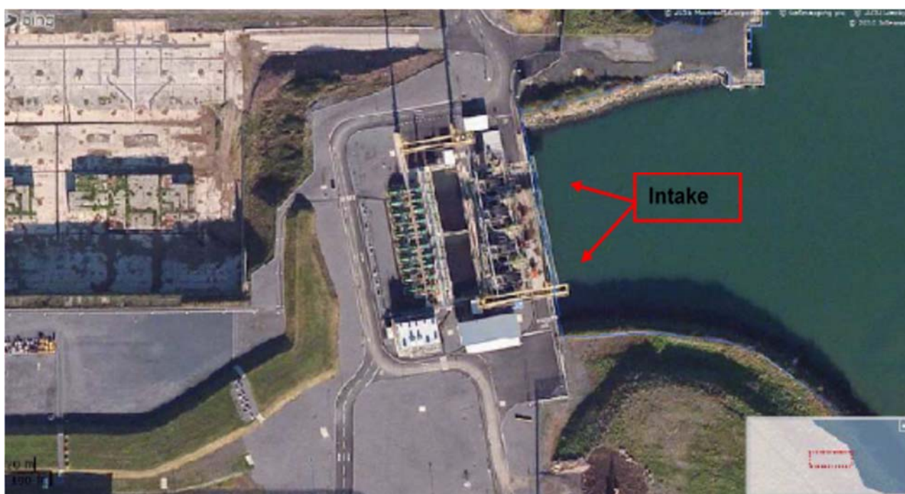
Figure 4.5 Aerial view of Pembroke CCGT
