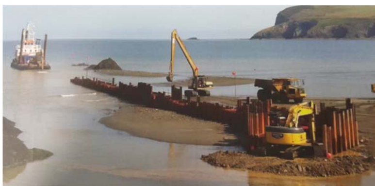
Figure 5.22 Photograph of conventional trench excavation and backfill operation.
