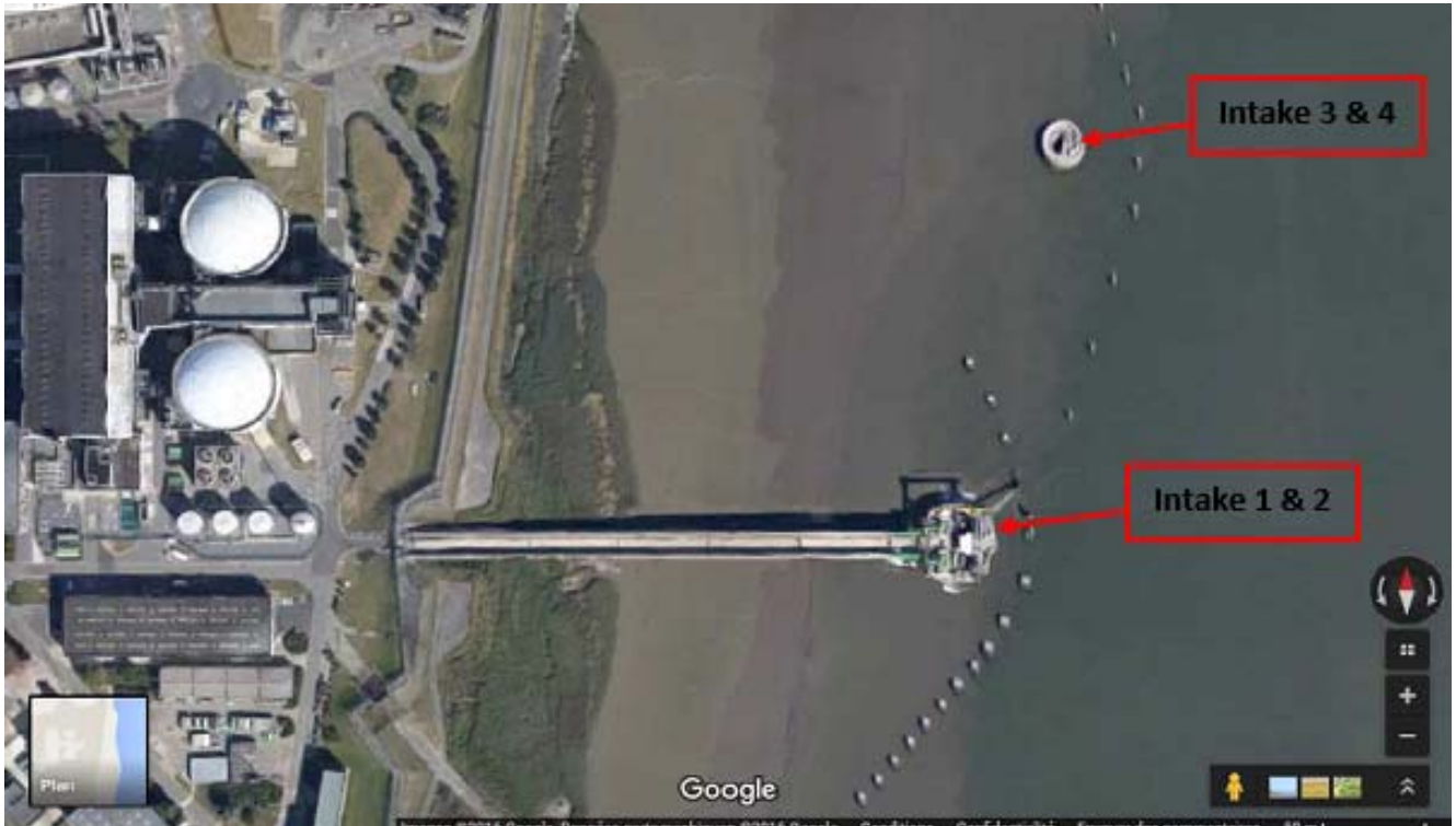
Figure 4.3 Aerial photograph of DOEL NPP on the Scheldt Estuary near Antwerp, Belgium, showing location of the water intake structures
