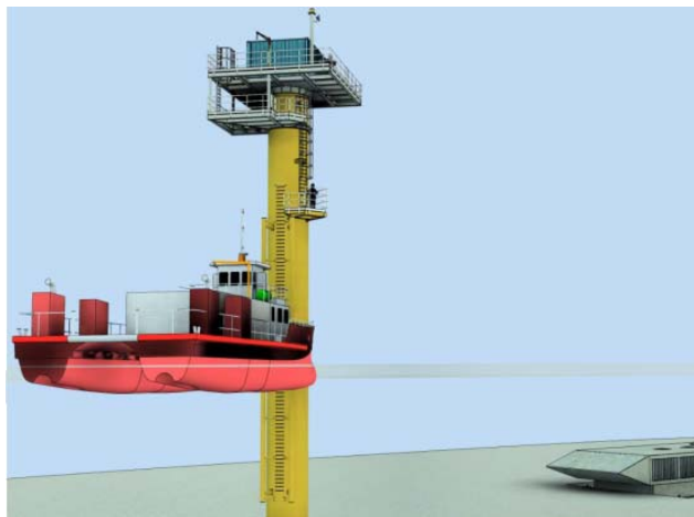
Figure 5.21 Depiction of a monopole central hub with transformer housed on a platform.
