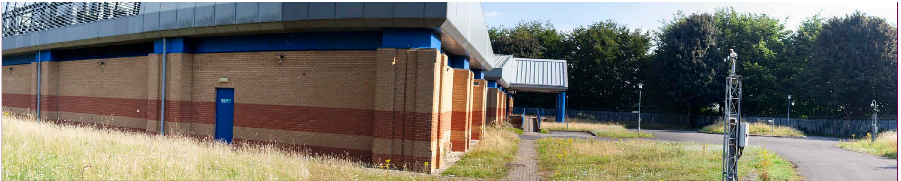
Viewpoint C8a: View north east of eastern data centre within secure fence.
