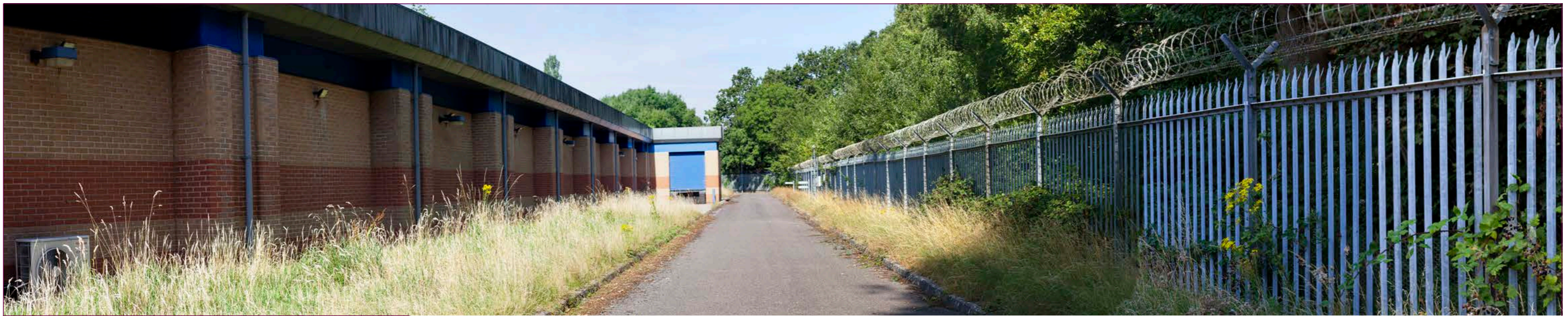
Viewpoint C9b: View north west along perimeter fence of eastern data centre.
