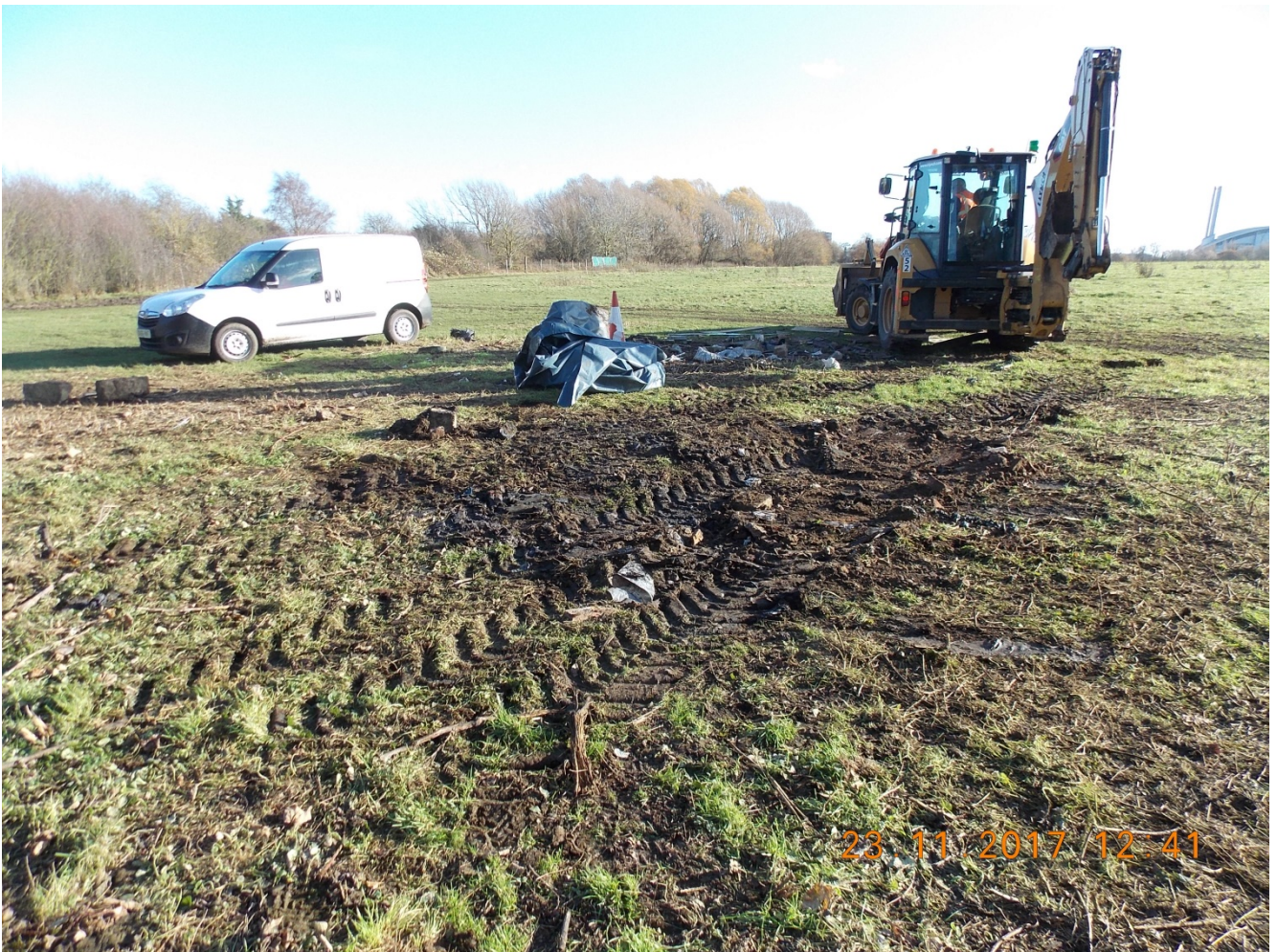
HEP-TT-9 (Post Condition)
