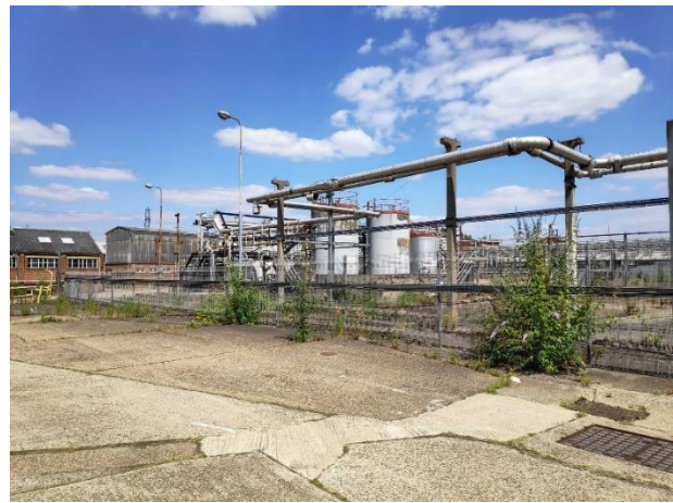
Plate 5.2: Piping structures and hardstanding in eastern section of the site
