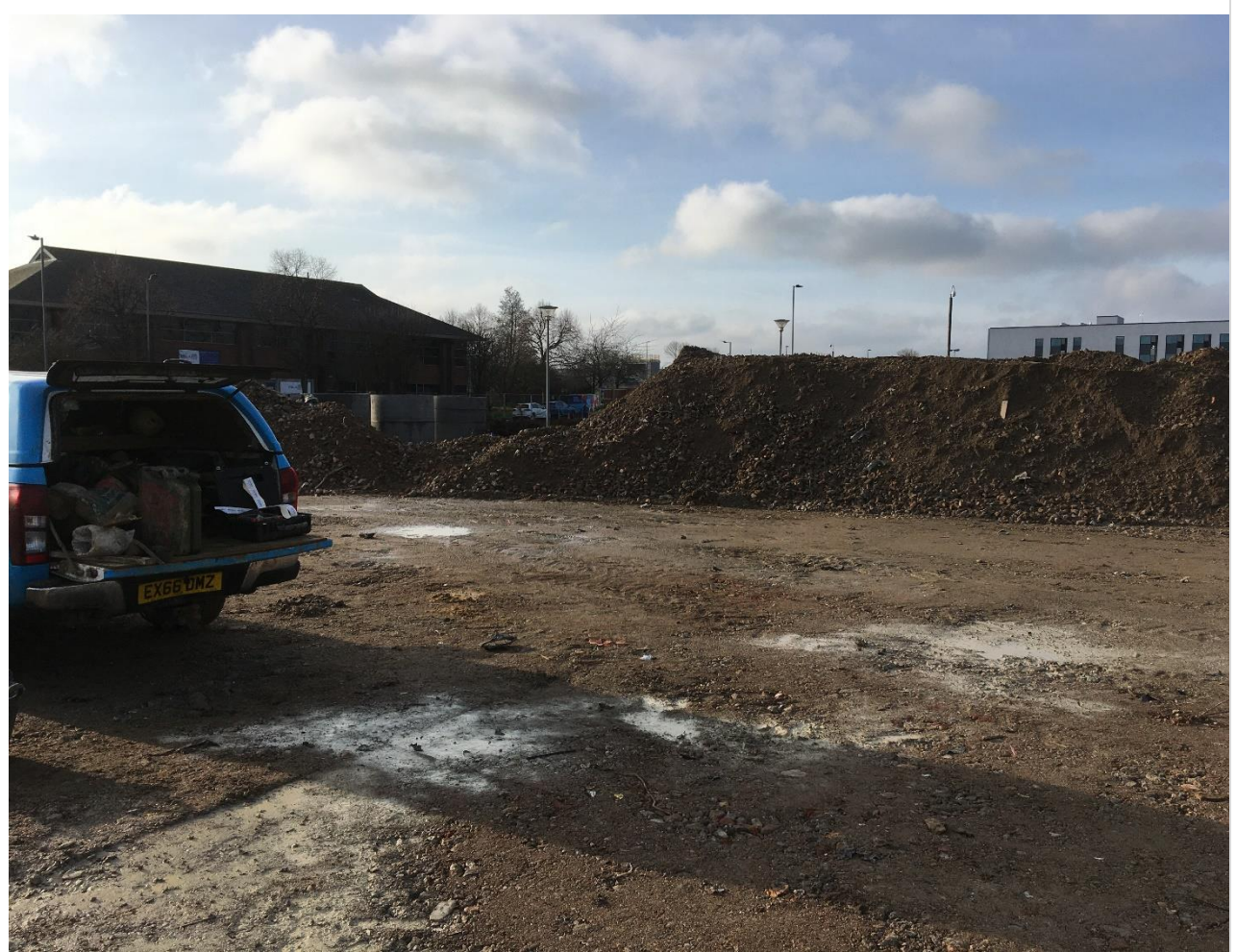
Photograph 6 – south west of site (post levelling/rolling)
