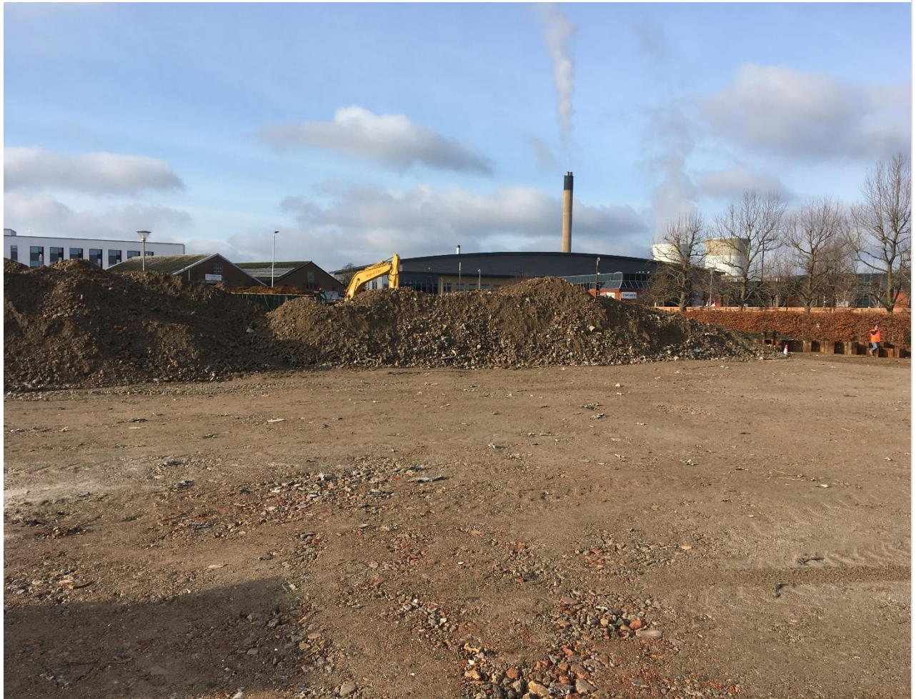
Photograph 7 – central west of site (post levelling/rolling)
