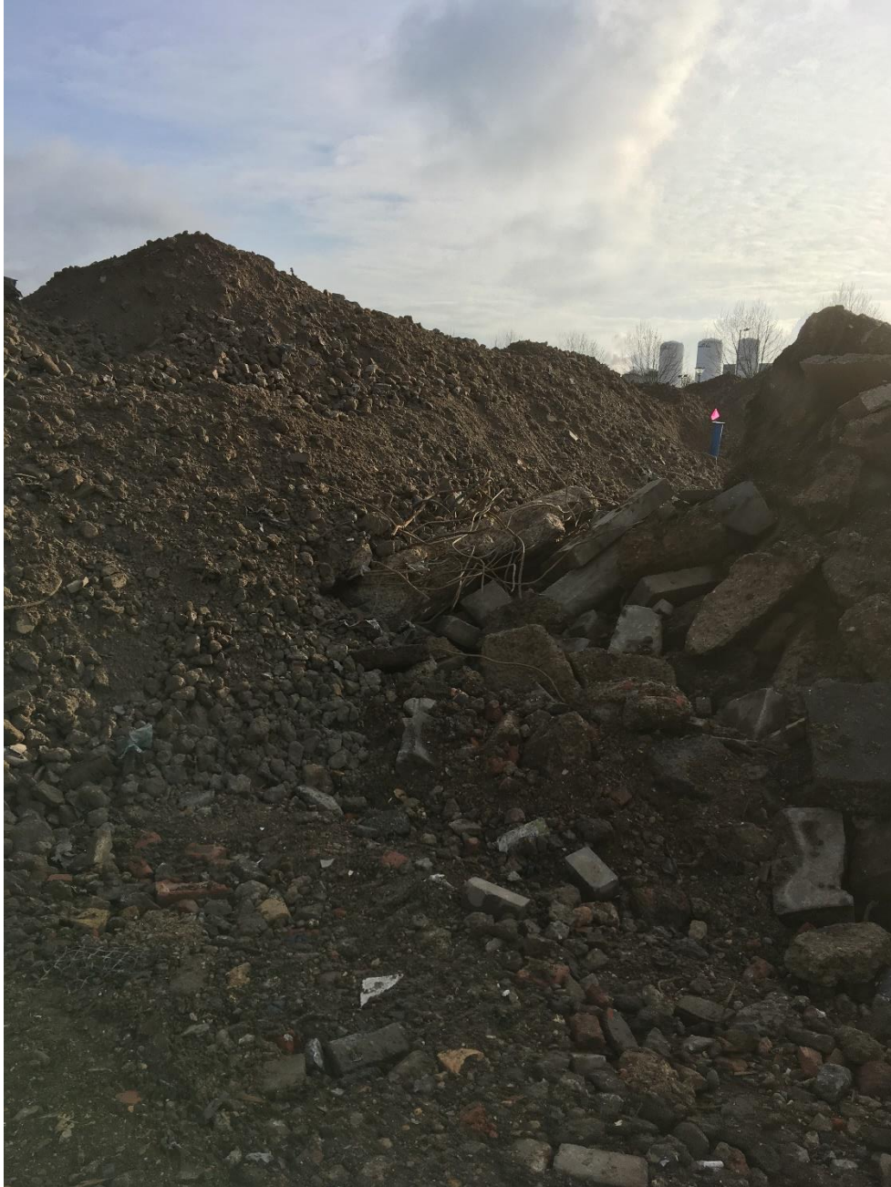
Photograph 15 – Residual demolition material from levelling stockpiled in the central west
