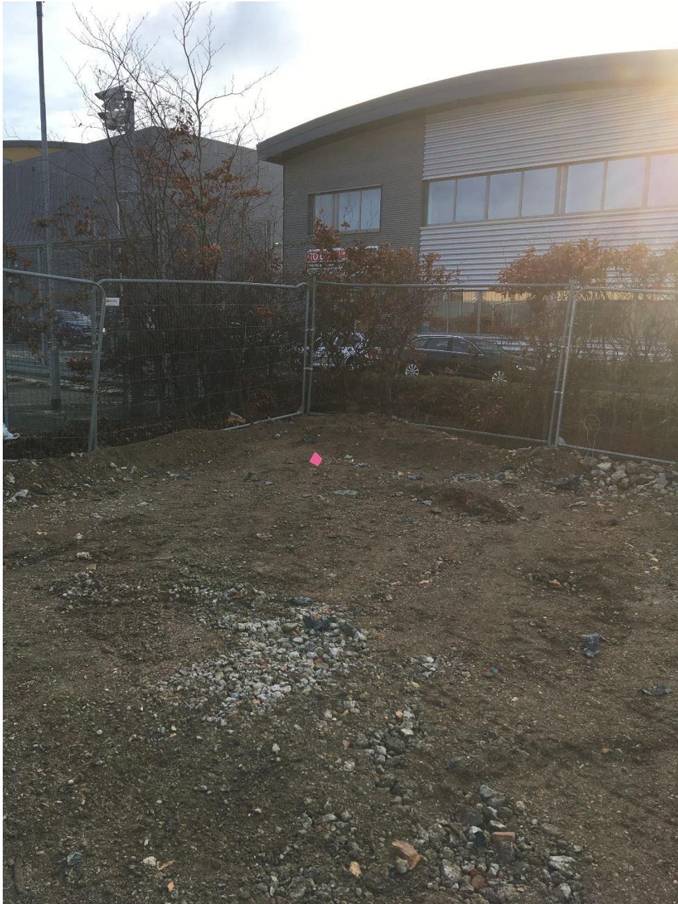
Photograph 17 – South East corner of Site (DS208)
