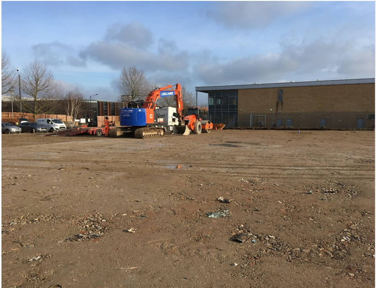
Photograph 4 – north east of site (post levelling/rolling)
