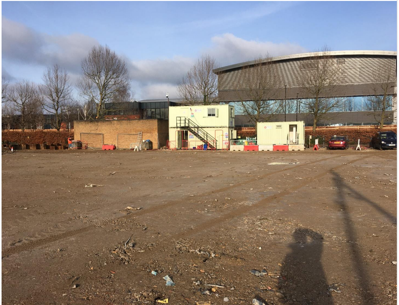
Photograph 8 – North of site (post levelling/rolling) substation and welfare.
