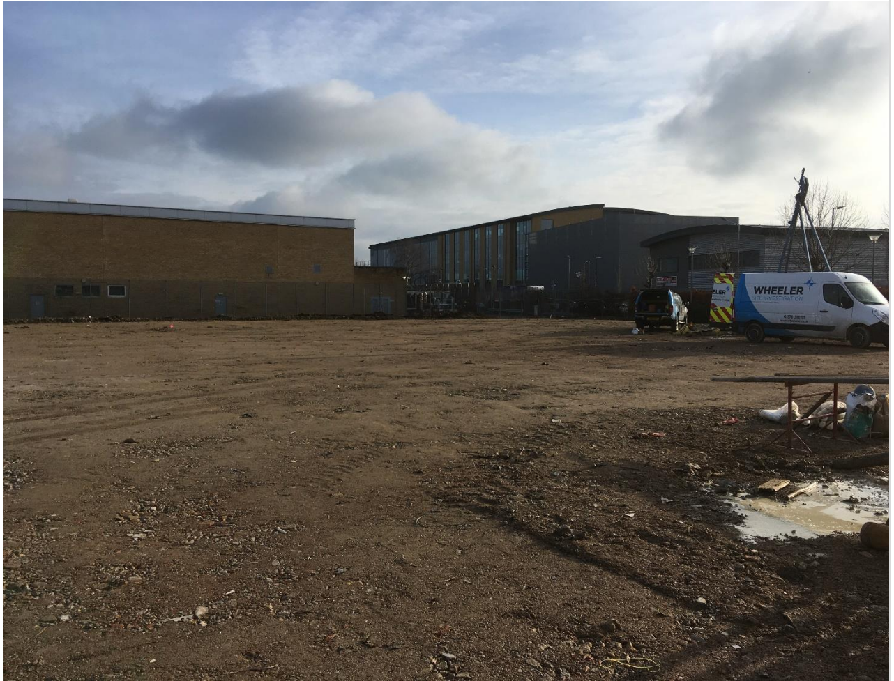
Photograph 5 – south east of site (post levelling/rolling)
