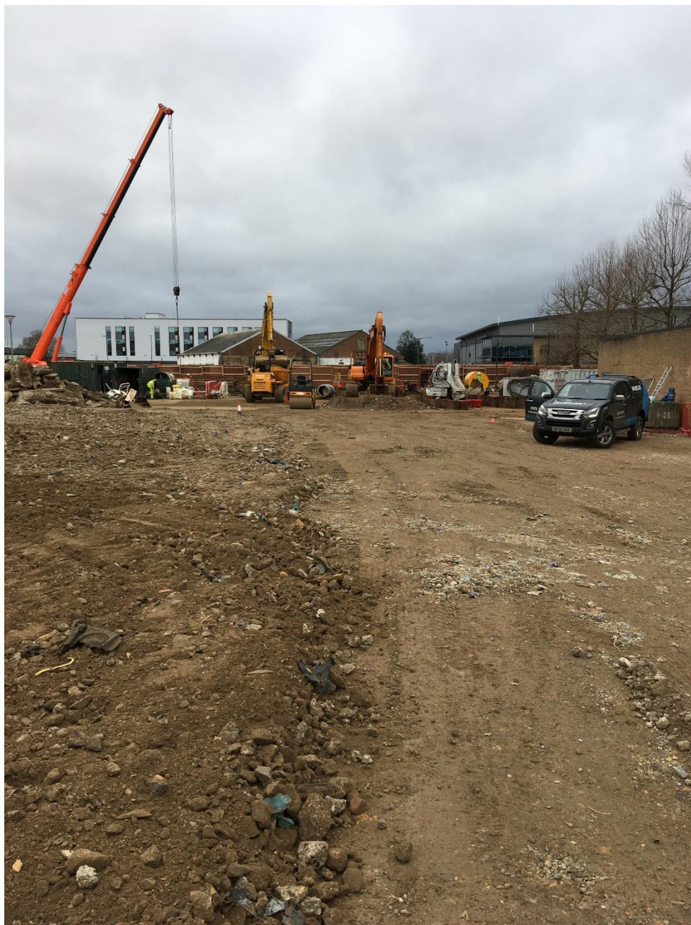
Photograph 1 – North west of site – Thames Water sewer diversion
