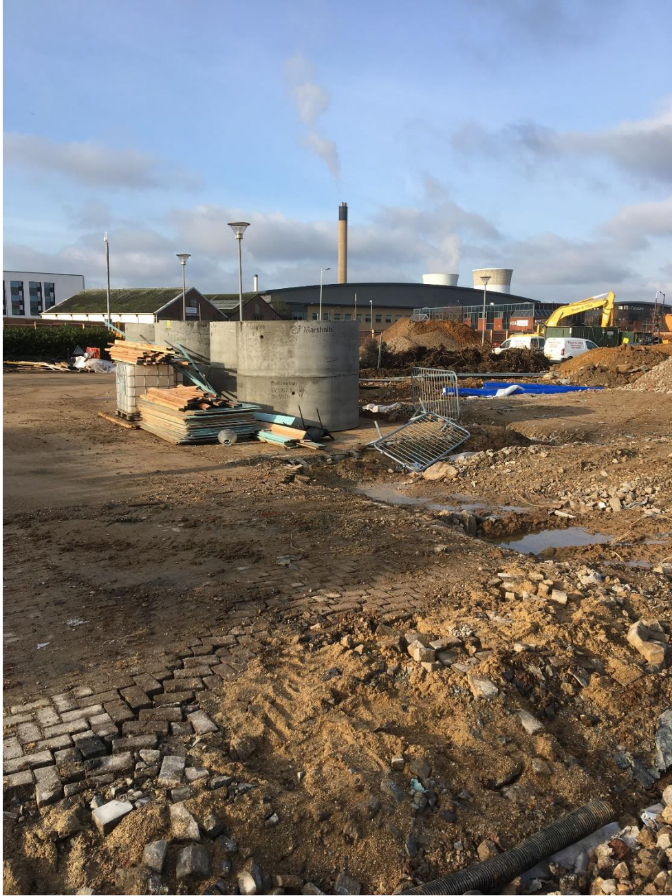
Photograph 10 –Thames Water sewer diversion works area
