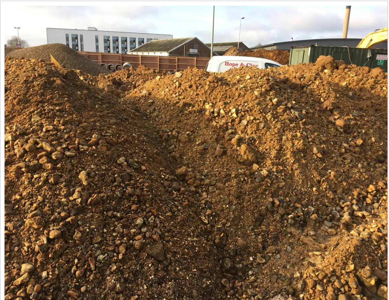
Photograph 12 – Taplow Gravel Formation removed for the Thames Water sewer diversion.
