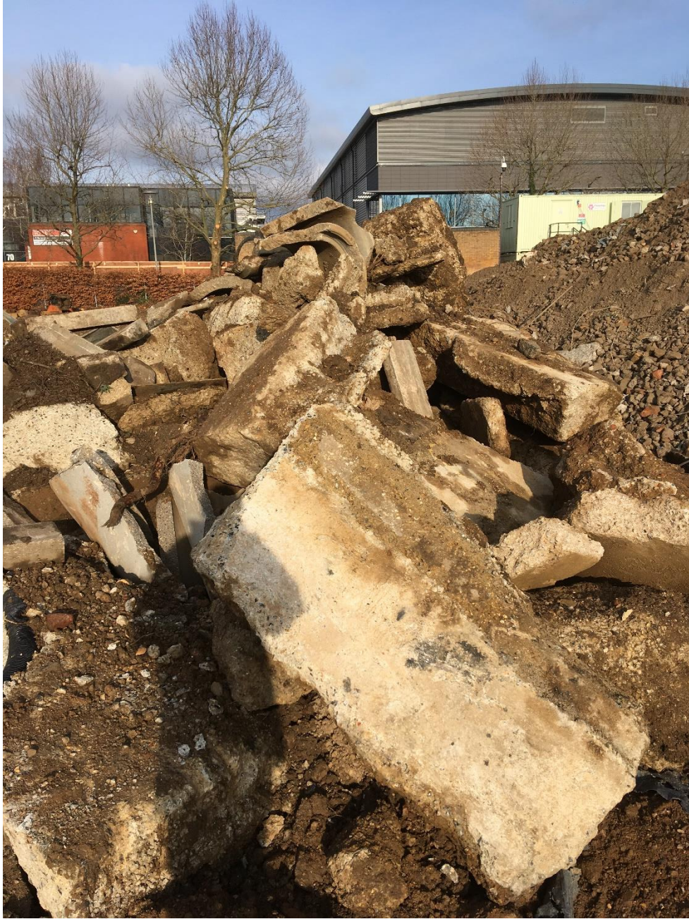
Photograph 14 – Large concrete foundations from demolition
