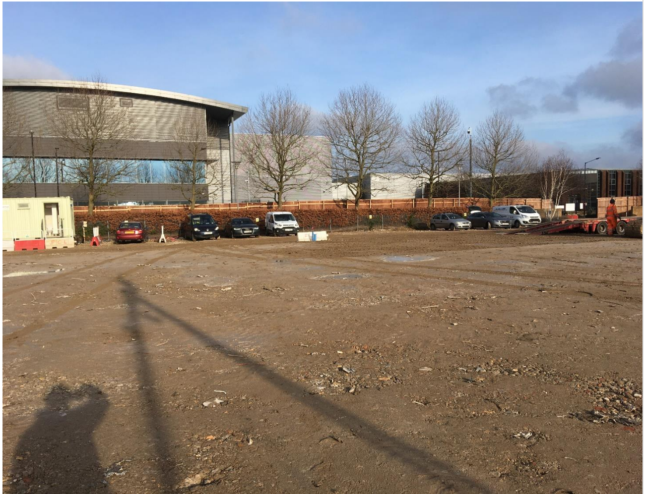
Photograph 9 – North east of site (post levelling/rolling)
