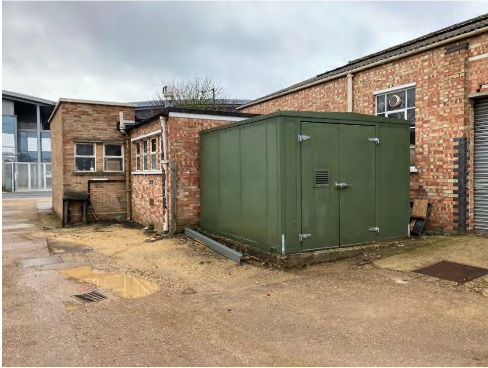
Photograph 11 – Unknown outbuilding in 660 Ajax Avenue external areas
