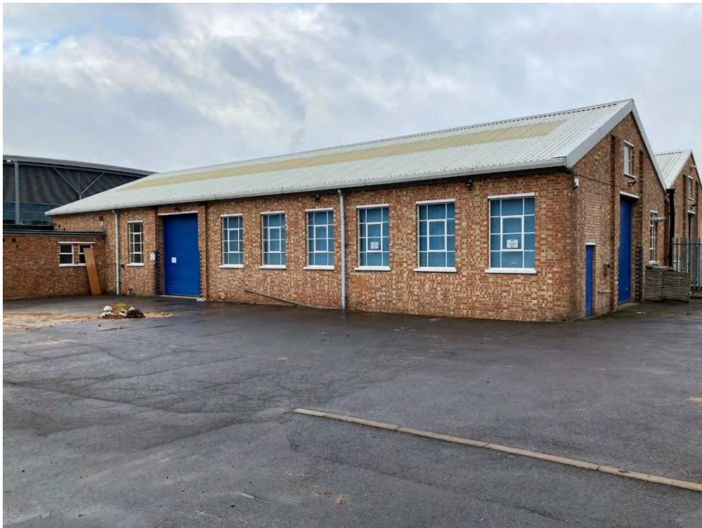
Photograph 8 – Typical brick warehouse (656 Ajax Avenue) with windows and corrugated iron roofing. External yard area laid to tarmac
