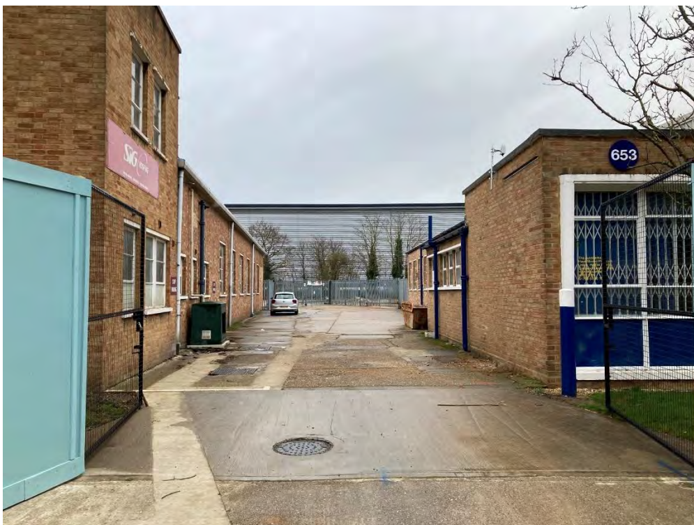
Photograph 2 – Typical access route into the Site's untenanted external yard areas
