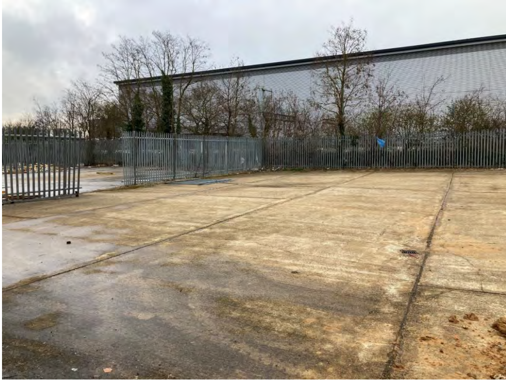
Photograph 5 – Typical yard area (654 Ajax Avenue) laid to concrete with metal fencing subdividing properties
