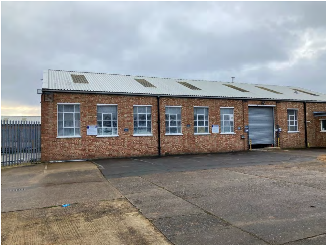
Photograph 6 – Typical brick warehouse (655 Ajax Avenue) with windows and corrugated iron roofing
