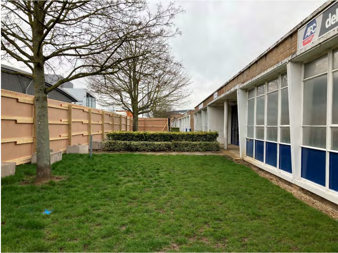
Photograph 9 – Soft landscaping along Ajax Avenue frontage
