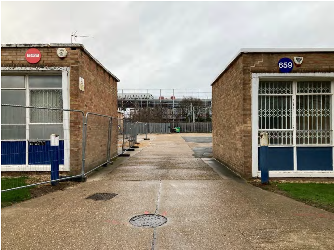
Photograph 10 – Entrance into 659 Ajax Avenue
