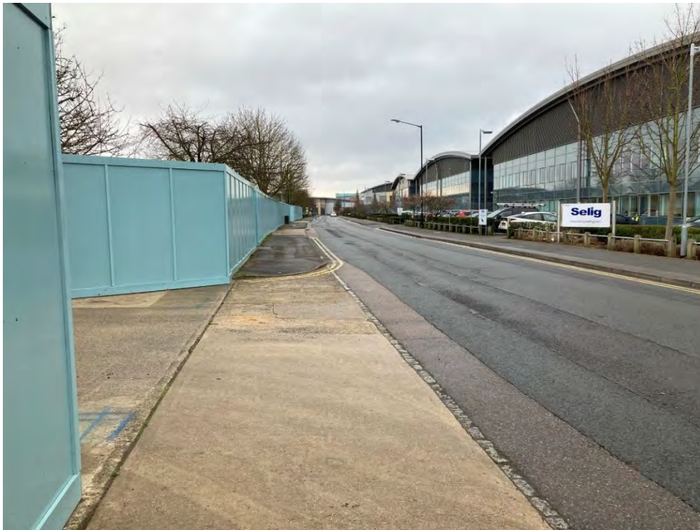
Photograph 1 – View of Ajax Avenue and light blue hoarding fence panels preventing access to 651-658 Ajax Avenue
