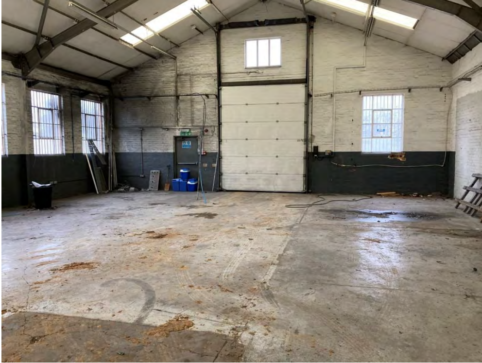
Photograph 3 – Typical internal warehouses at the Site with electronic roller shutters (653 Ajax Avenue)
