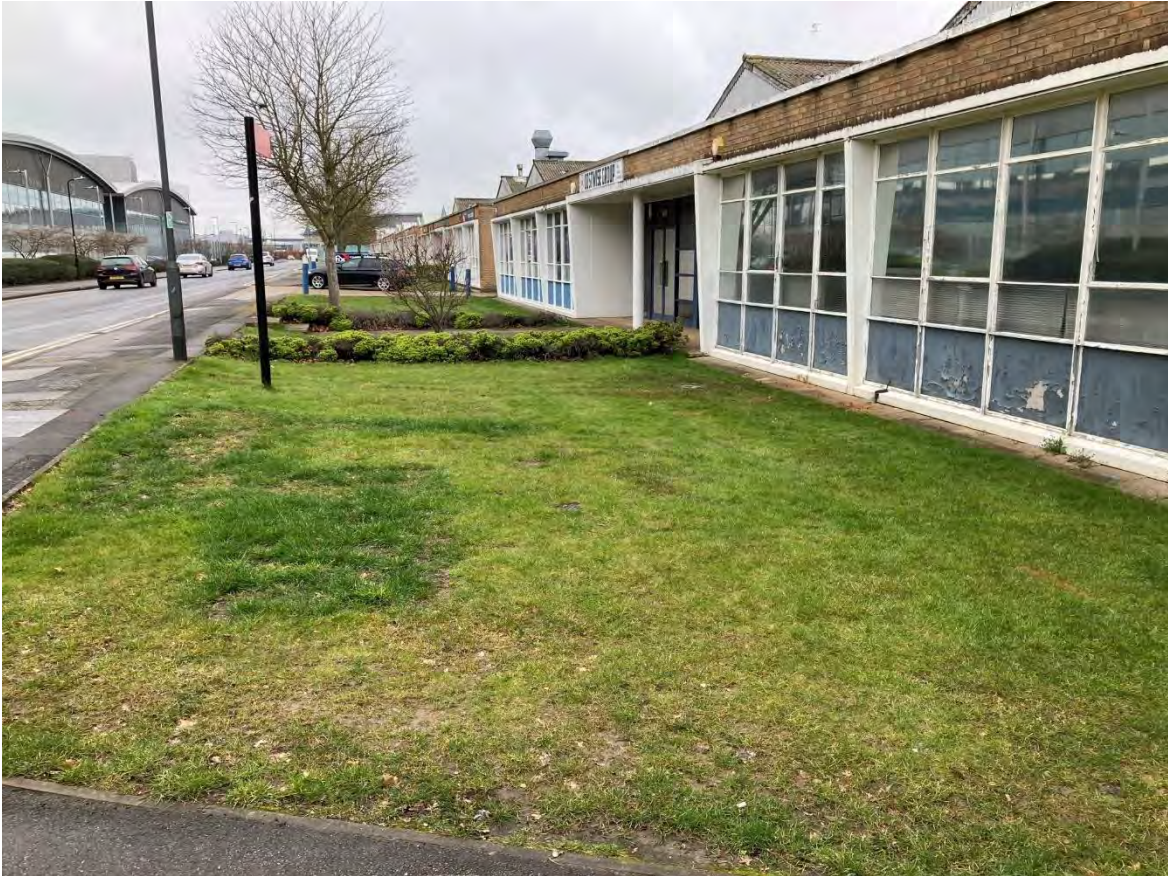
Photograph 13 – Soft landscaping along Ajax Avenue frontage
