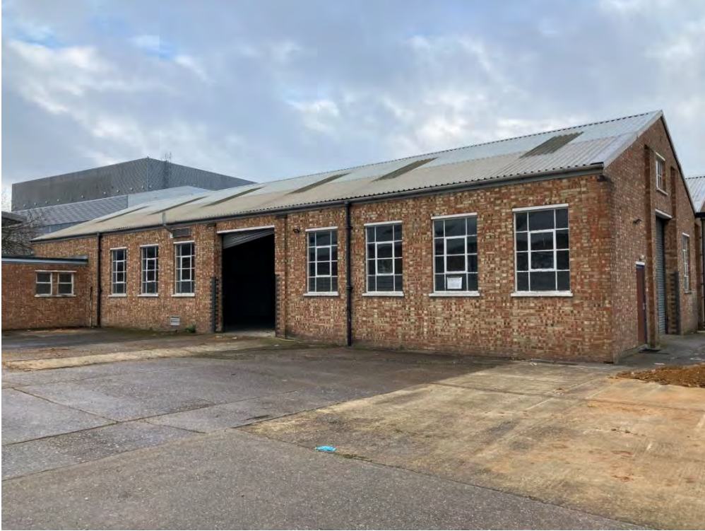
Photograph 7 – Typical brick warehouse (654 Ajax Avenue) with windows and corrugated iron roofing.
