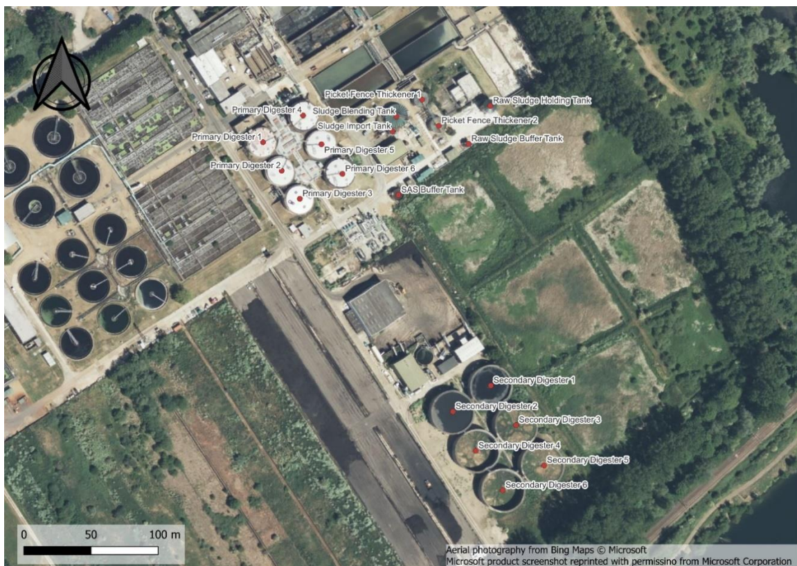
Figure 2-3 Labelled image of the assets within Rye Meads STW
