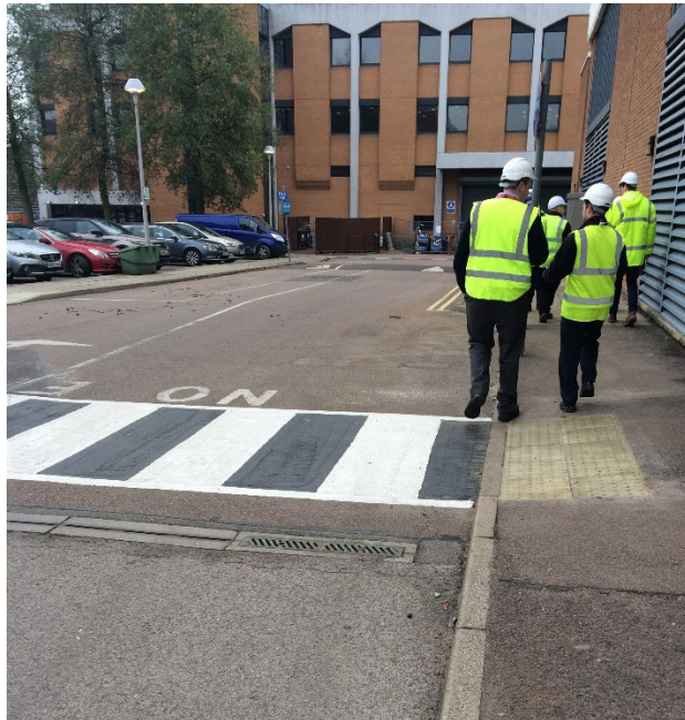
Photo 6. Roadway and surface falls adjacent to offset fill point to bulk fuel tank
