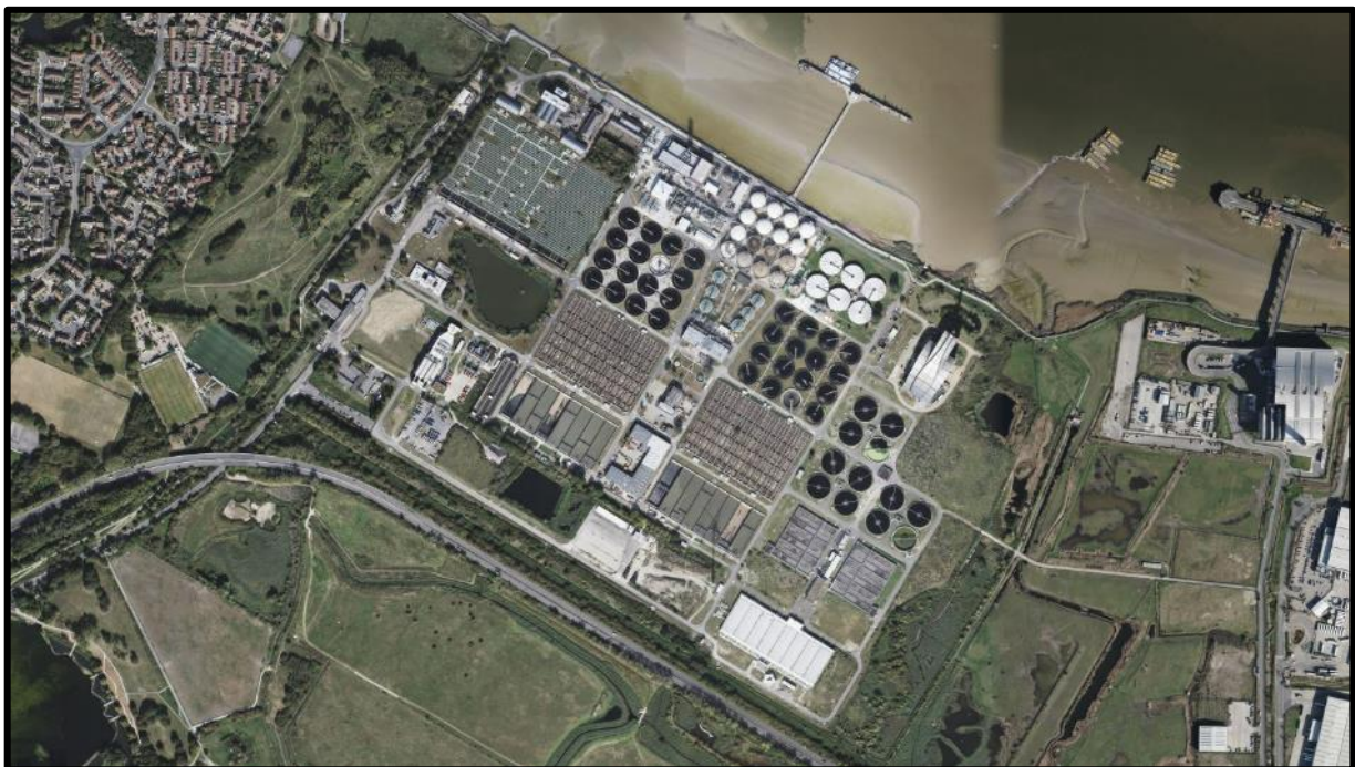
Figure 2-2 – Aerial Image of Crossness Sewage Treatment Works
