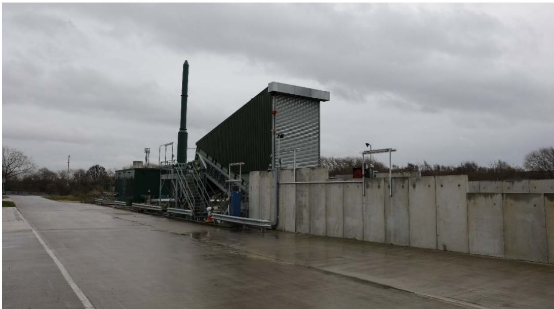
Figure F Dedicated sludge cake reception area
