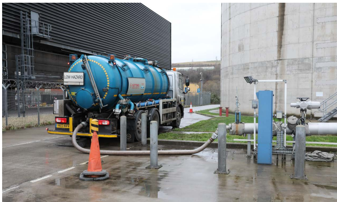
Figure D Sludge unloading via WaSP loggers
