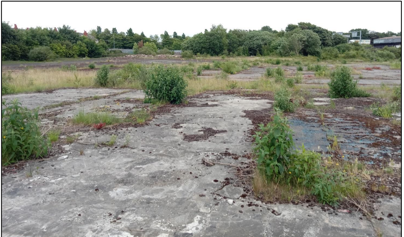
Plate 6 View of north eastern area looking roughly north east
