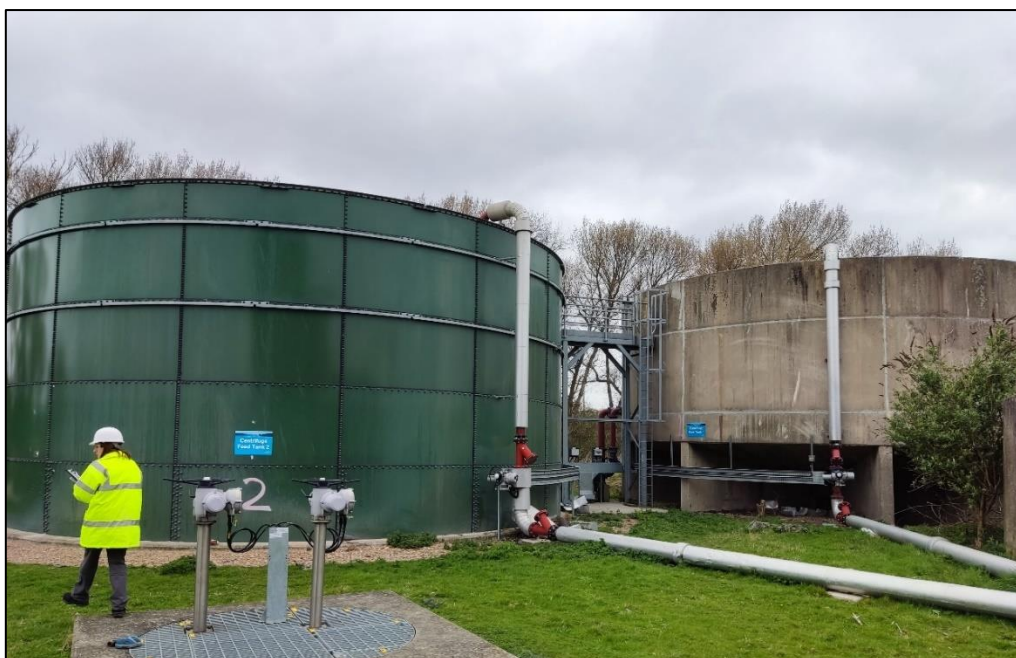
Figure 14. Centrifuge feed tank (no. 1 on the right, no. 2 on the left).
