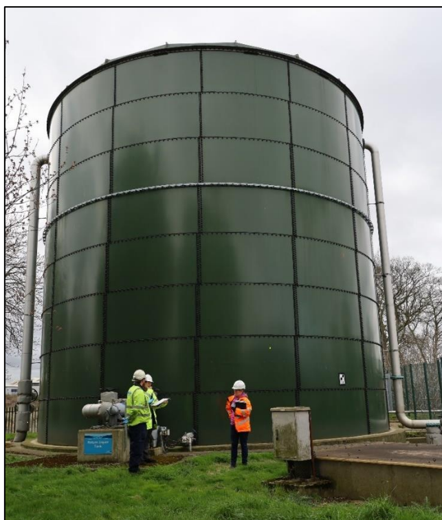
Figure 16. Return liquor balance tank
