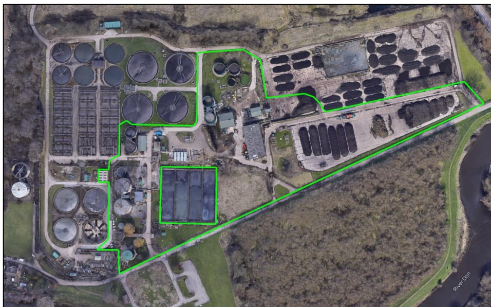
Figure 1. Aldwarke STF aerial view, installation boundary in green. © Google, 2021
