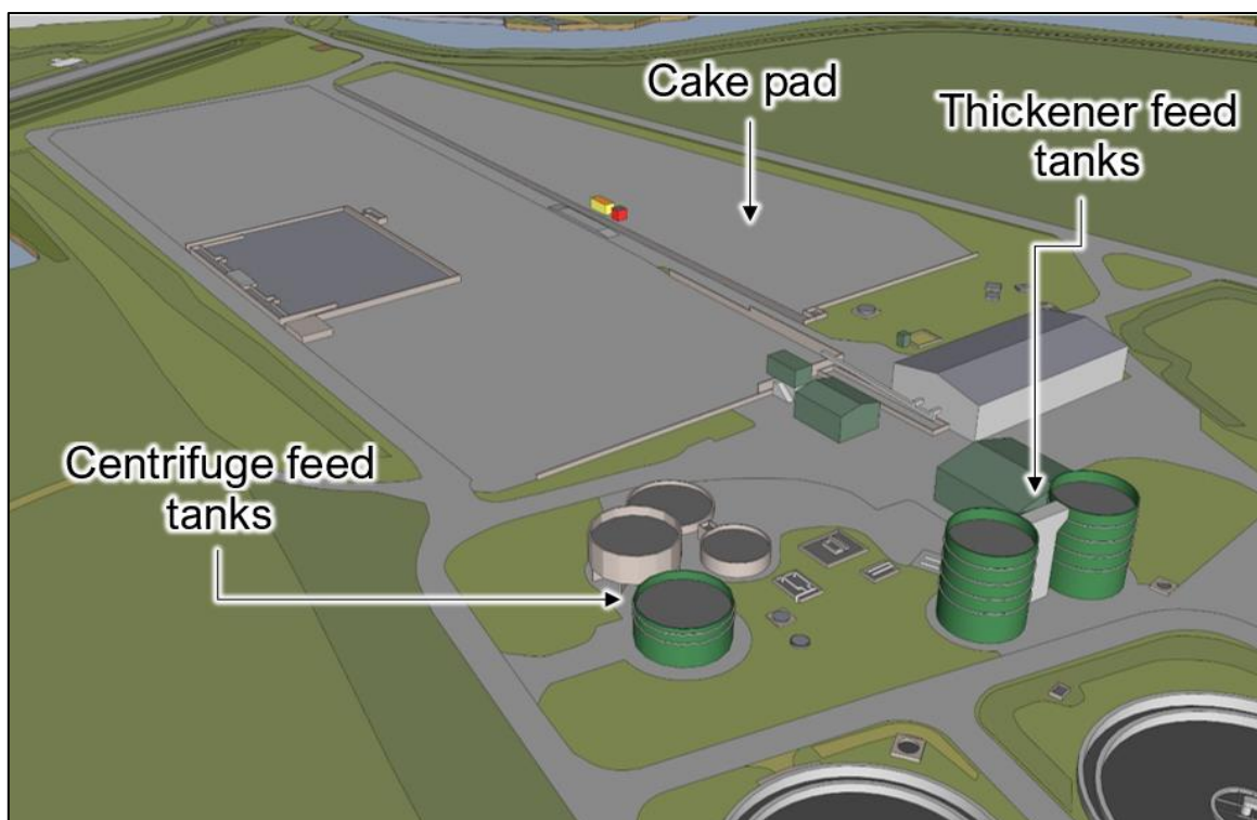
Figure 7. Sludge vessels located in the central north section of the site (view 1).
