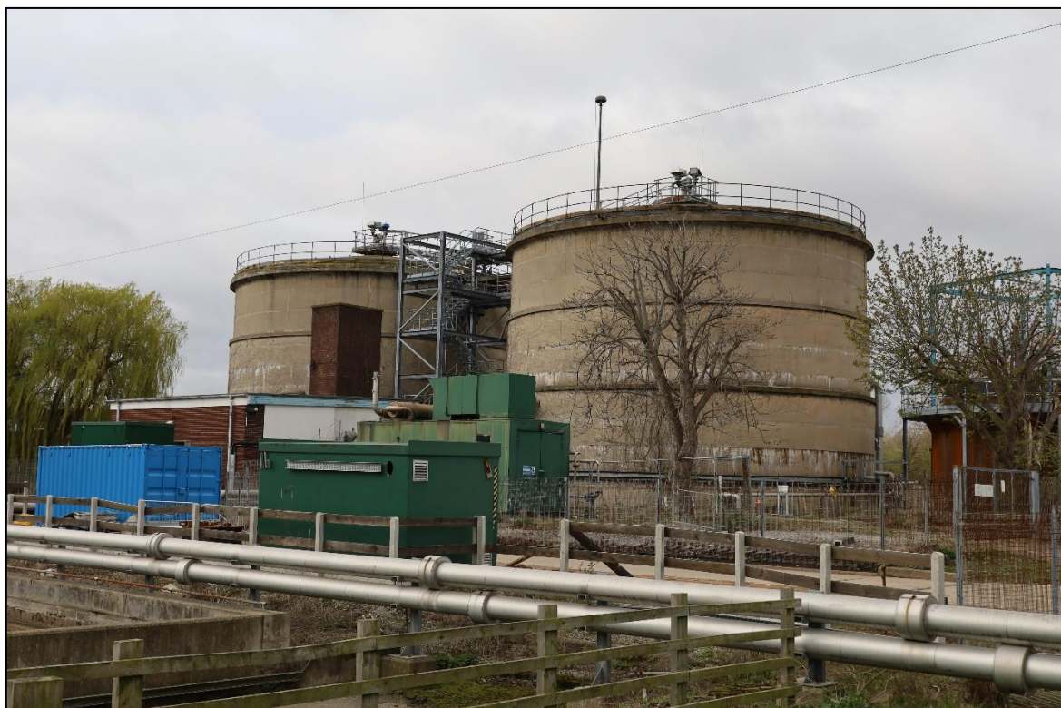
Figure 13. Digesters (2 no.).
