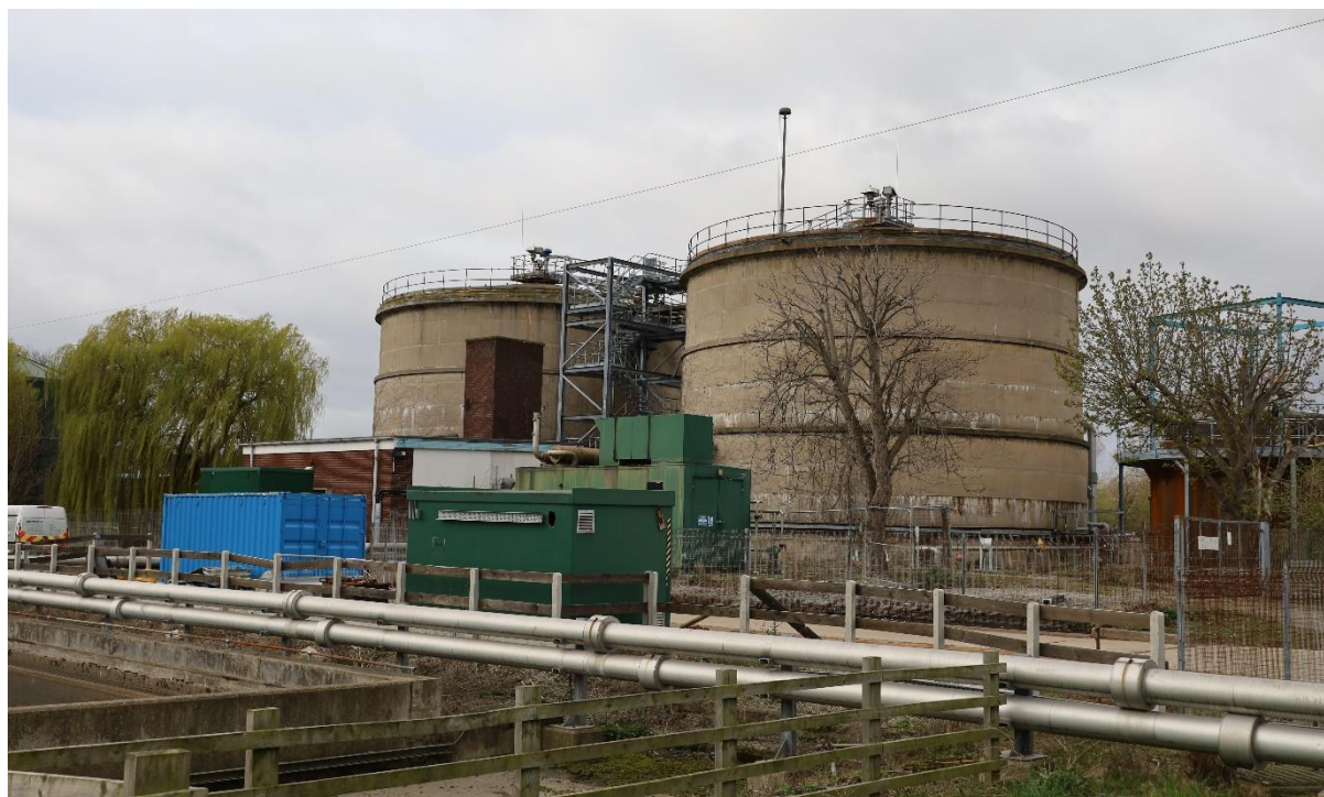
Figure I Digesters and CHP1
