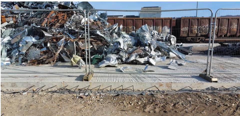
Photograph 6-2: Installation of new surfacing (Feb-2023)
