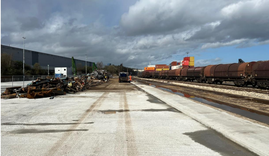
Photograph 6-5: Site surfacing, within the storage area, post-upgrade (March 2023)
