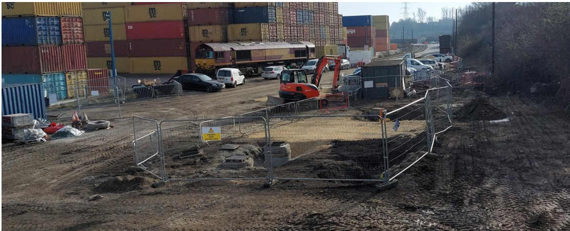
Photograph 6-1: Installation of infrastructure and manhole S14 (Feb-2023)
