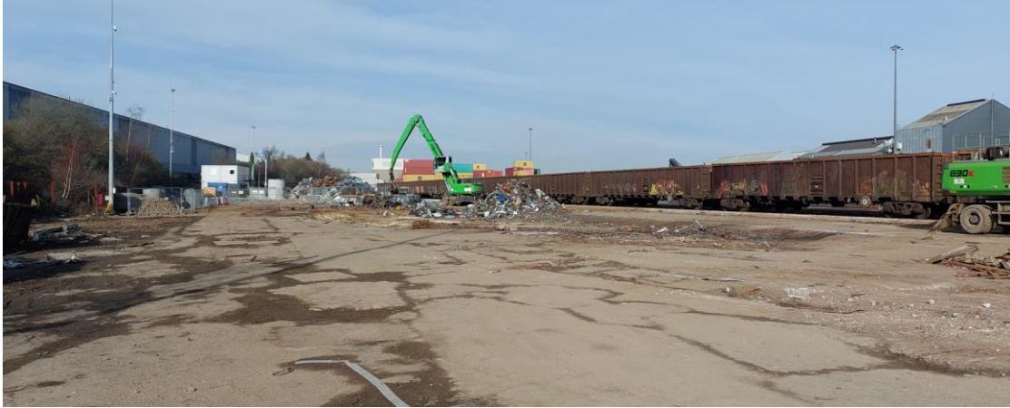
Photograph 6-3: Site surfacing before upgrade (February 2023)
