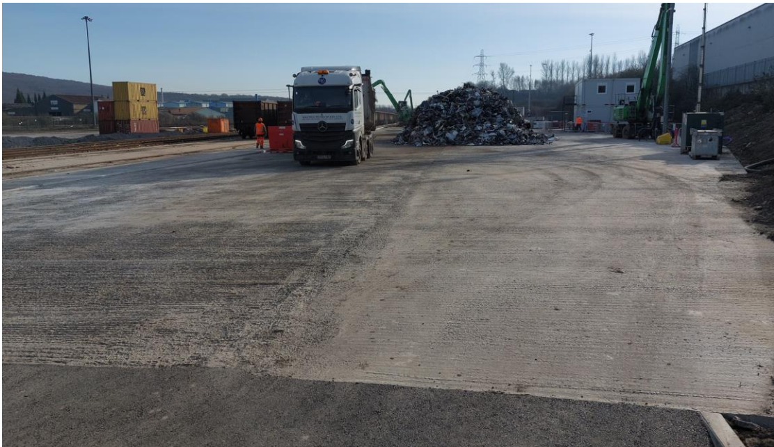
Photograph 6-4: Site surfacing, exit from internal road, post-upgrade (February 2023)
