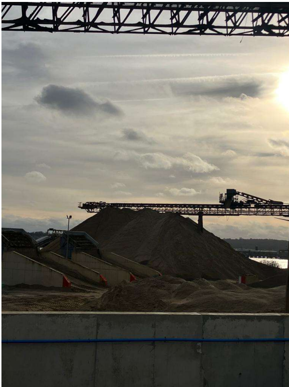
Photograph C – View showing towards the south showing stockpiles of material at the Hanson site.
