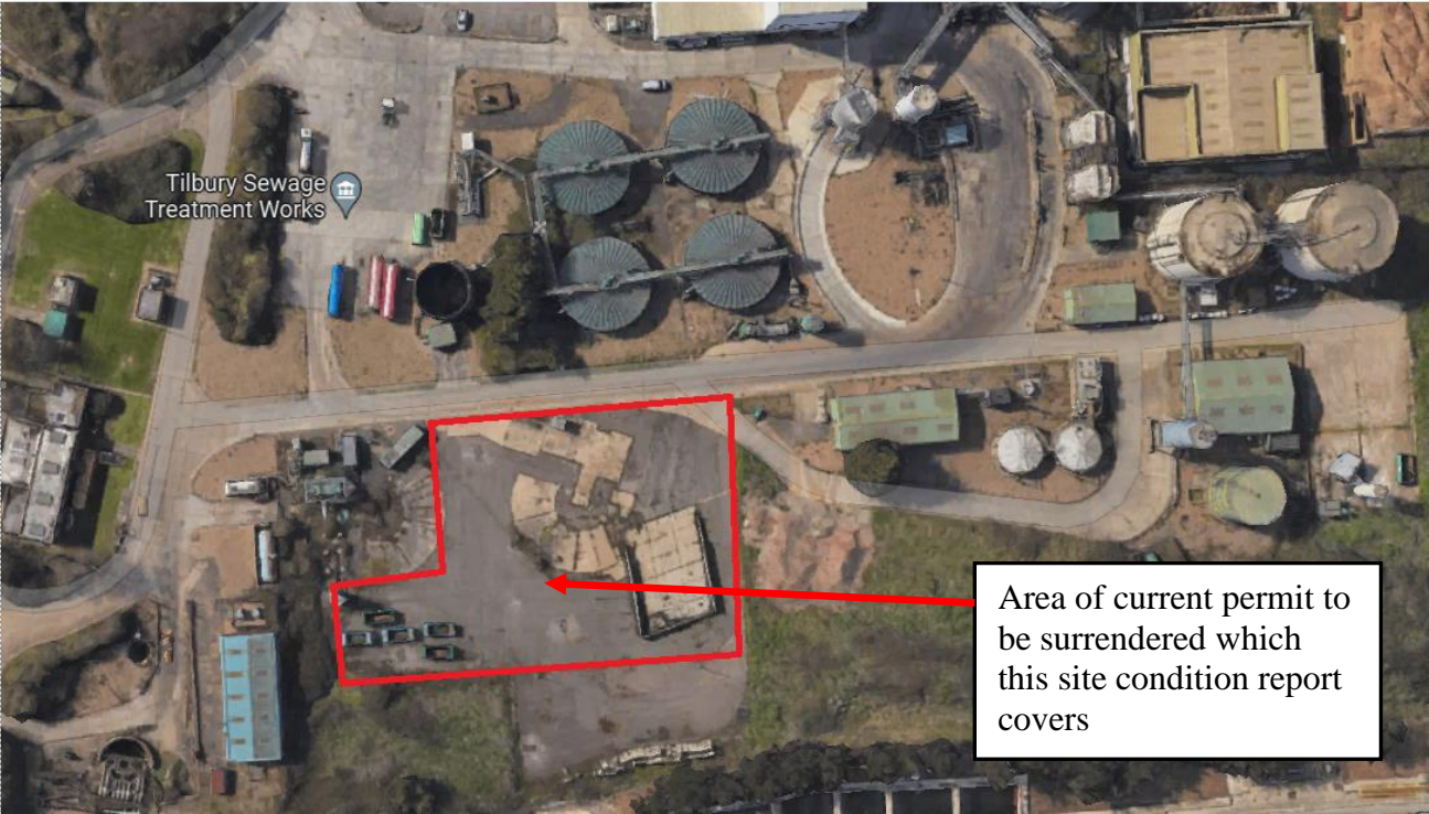
Figure 2: Tilbury Sludge Treatment Centre with red line boundary of permit area to be surrendered
