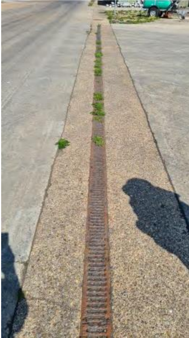
Photographs 3,4 and 5 showing the drainage at the western edge of the Storage area
