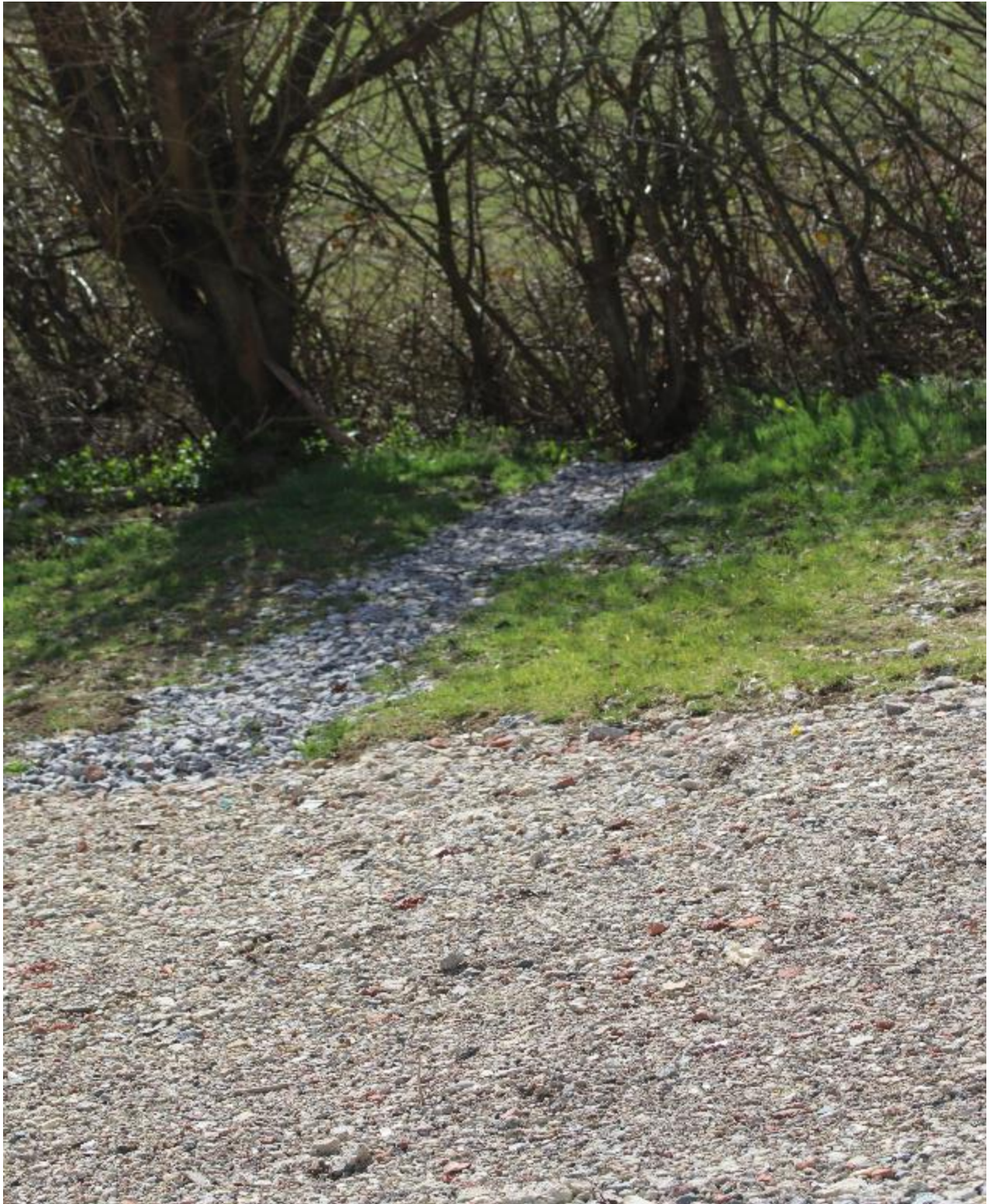
Picture 5 Stone covered pipe across roadway
