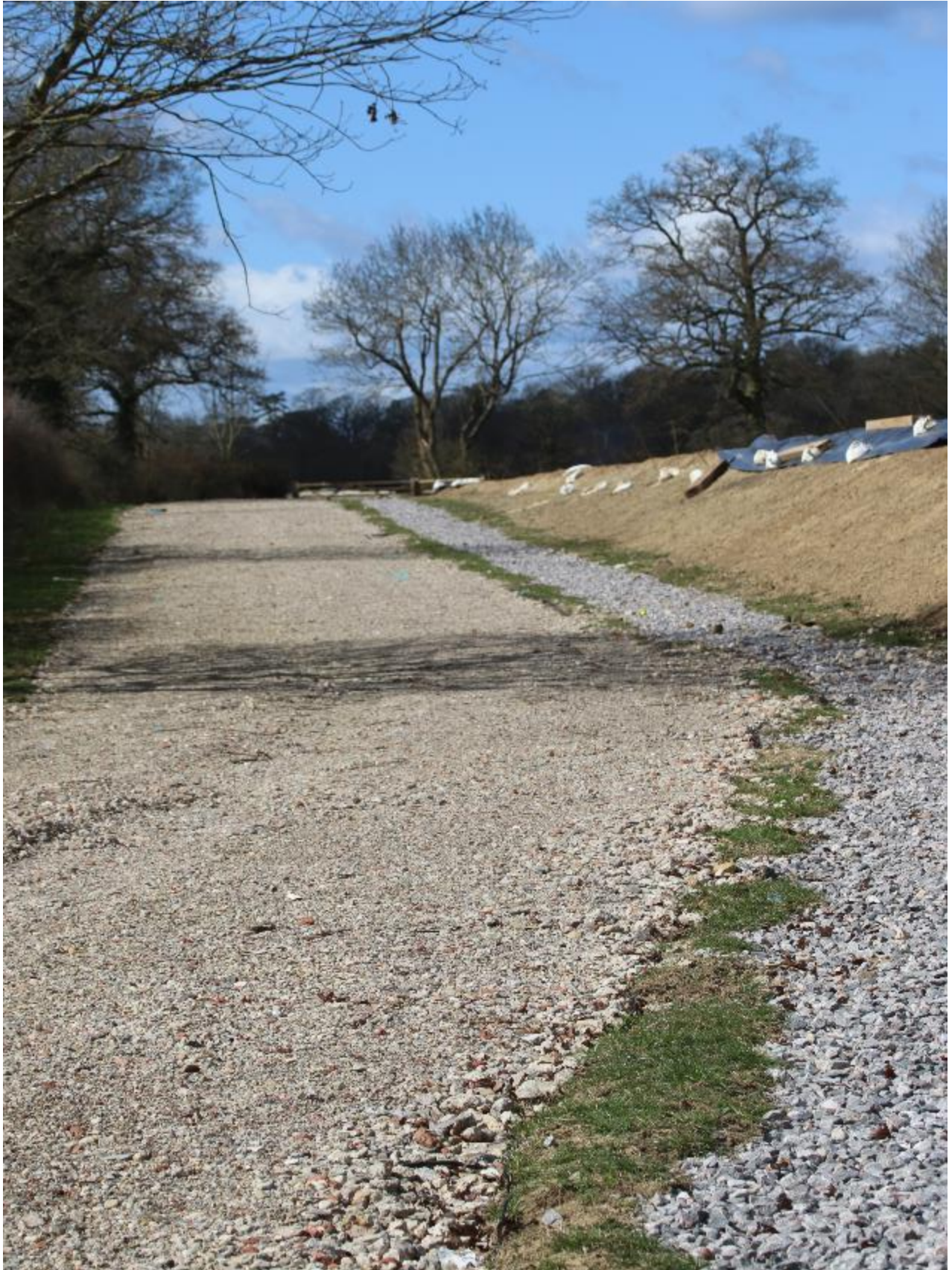
Picture 6 and 7 Stone covered pipe from separator to dyke
