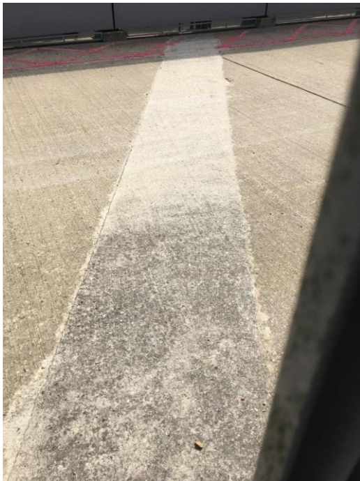
Figure 12: Unit 3 underground pipework marking
